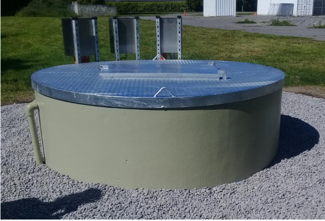
7. Installation of Secure, Accessible Well cover
