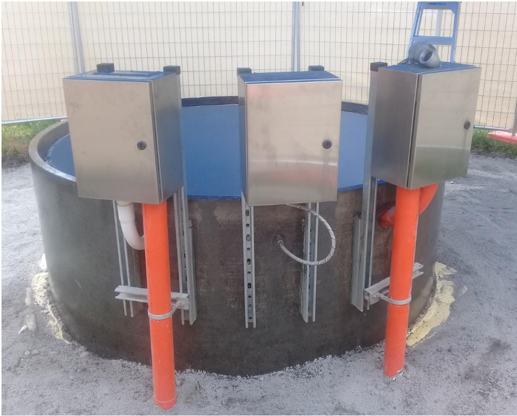
Ideal Picture (Main Pumps Well 2)
