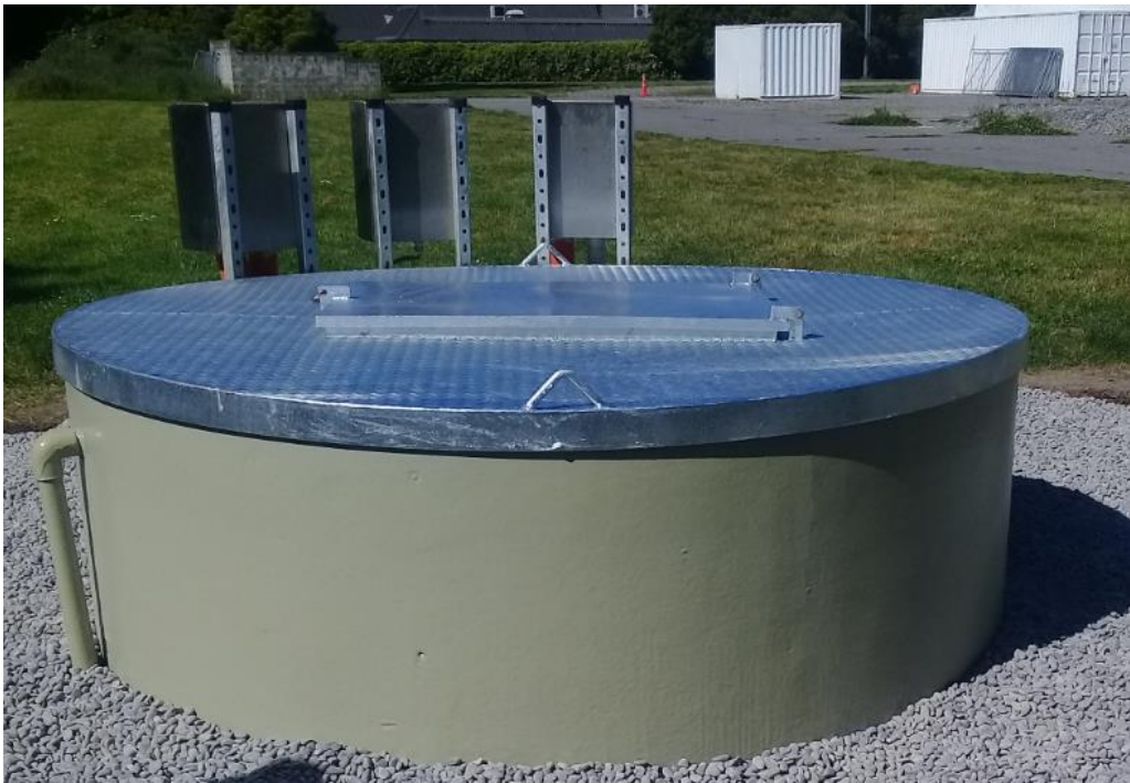
Ideal picture (Main Pumps Well 2)
