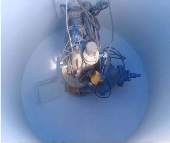
2/3.Internal Sealing and Lining of the Well
