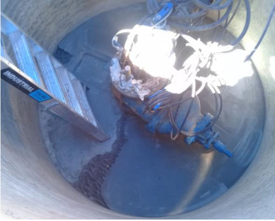
5/6. Floor Regrading (in progress)
