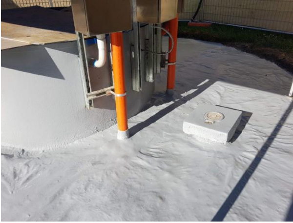
9.Construction of a 2m Apron around Well
