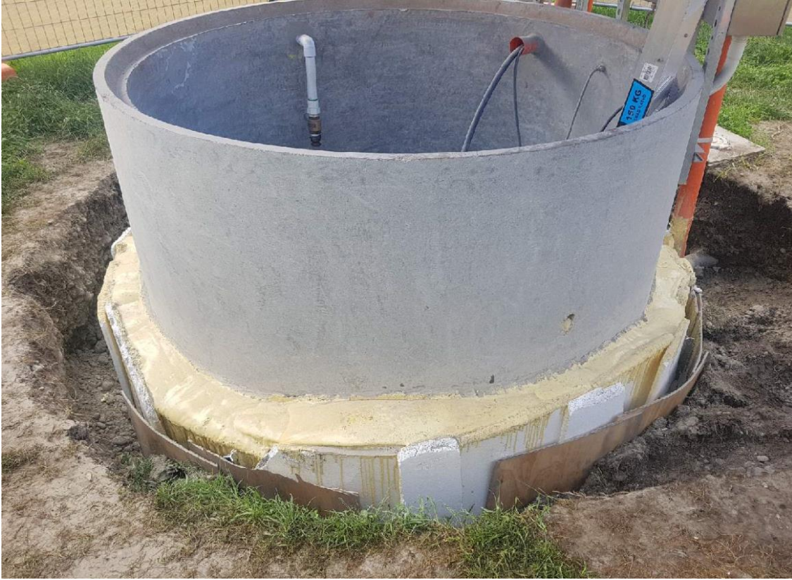
Ideal Well Picture (Main pumps Well 2)
