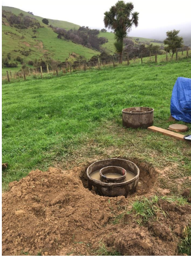
Photograph 5: Infiltration Test IT4 surface and subsurface within Robinsons Bay (Site 4).
