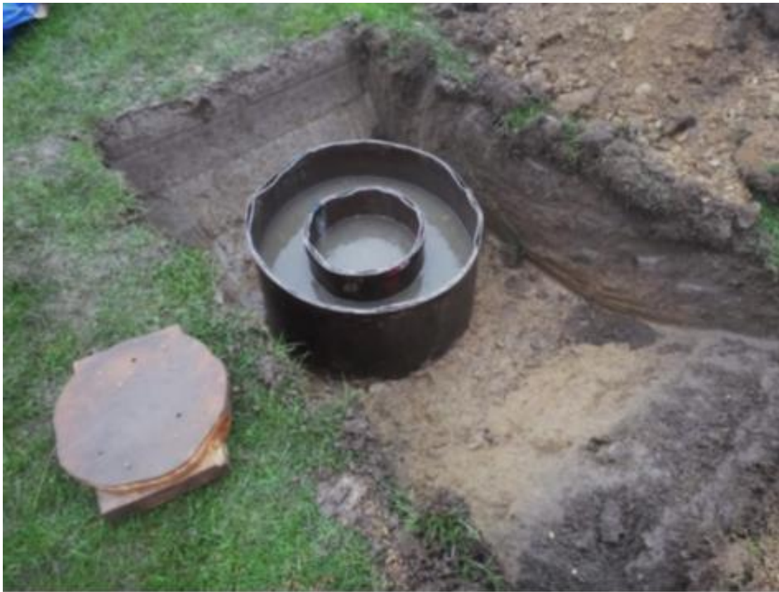
Photograph 10: Infiltration Test IT8 sub-surface test within Pompeys Pillar (Site 8).
