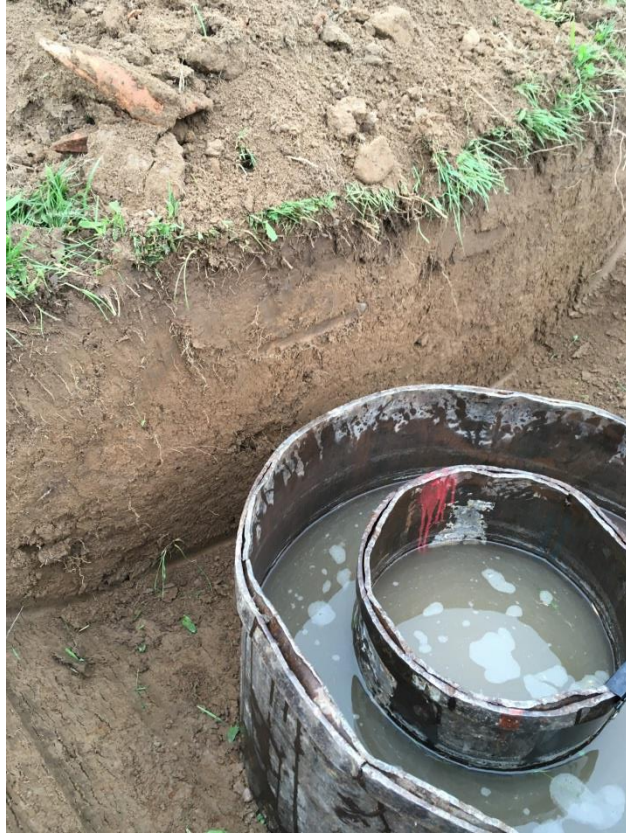
Photograph 3: Infiltration Test IT2 sub-surface infiltration test within Robinsons Bay (Site 2), surface test IT2 not shown..
