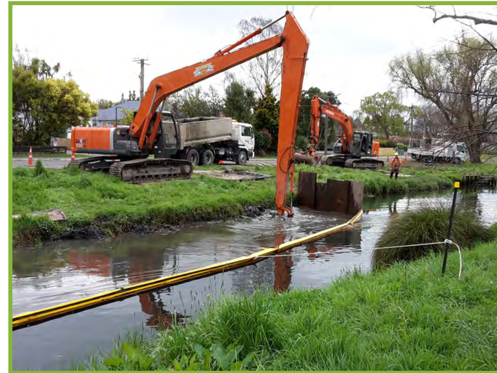
Silt removal in the Heathcote River.
