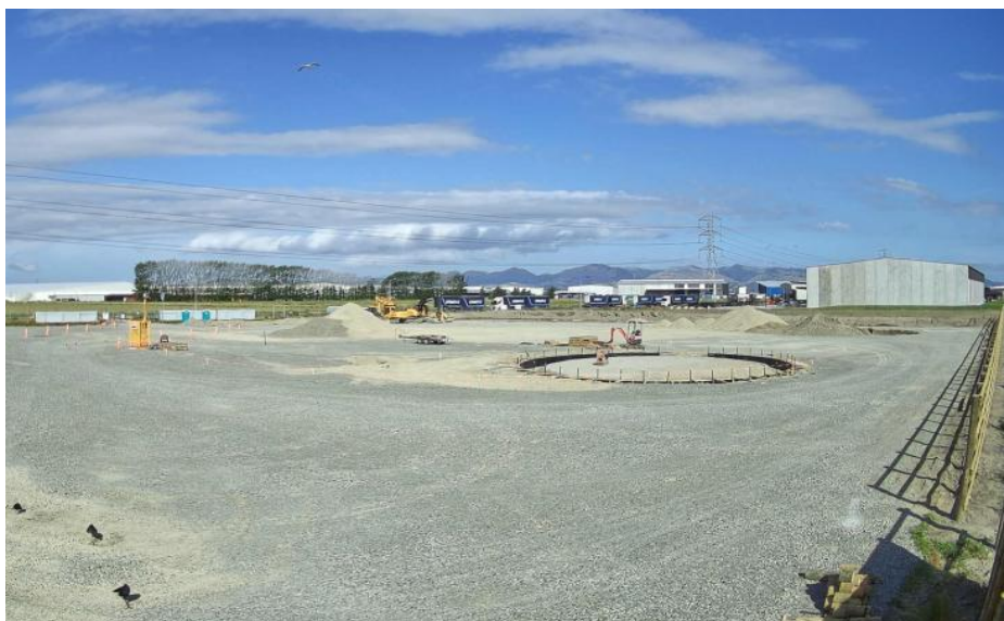
Foundation for the first hydrolysis tank, 19m in diameter
