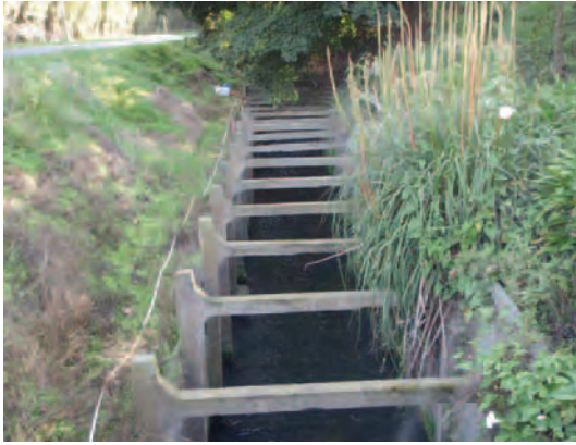
Site 12: Horner's Drain (looking downstream from top of site)
