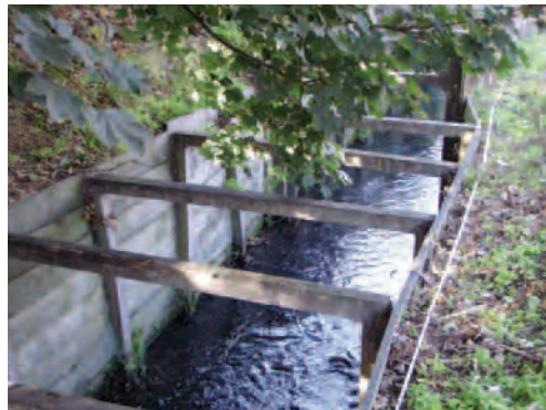
Site 12 (ranked 15th equal), Horner's Drain, looking upstream
