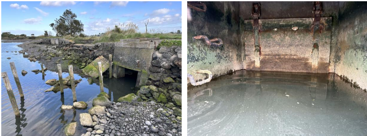
Figure 6: The culvert outlet of Charlesworth Drain (left) and internal flap gate (right), during the October 2024 visit (incoming tide).
