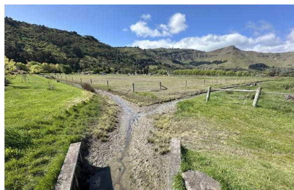
Structure 5: Munning Habitat
