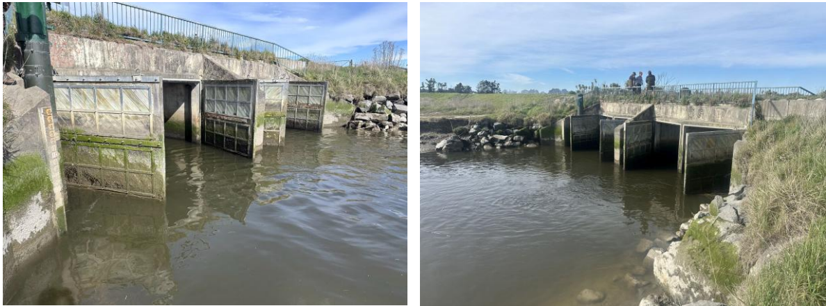
Figure 2: The tide gates in the Styx River, near the outlet into Brooklands Lagoon.
