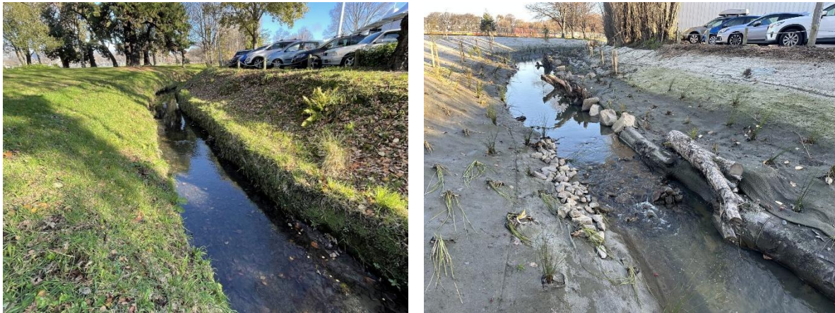
Figure 30: Addington Brook, in April 2022 prior to restoration (left) and immediately following restoration in June 2024 (right), showing bank battering the addition of wood and riffle habitat, and new native plantings.
