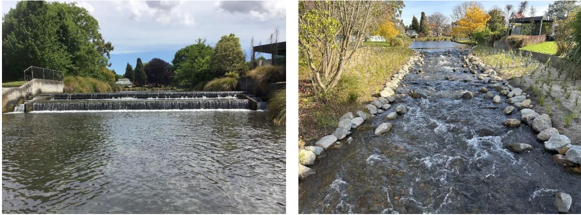
Figure 29: Mona Vale weir, in 2020 prior to remediation (left) and in 2023, after remediation to enhance fish passage (right).
