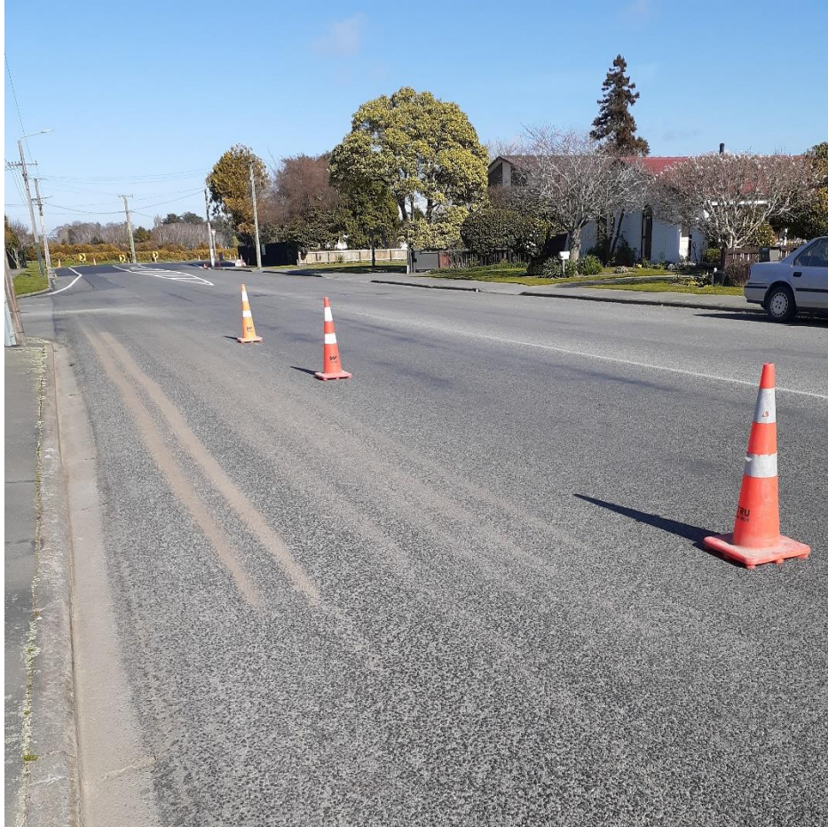
Figure 4-14: Dirt streaks on road created by regenerative sweeper
