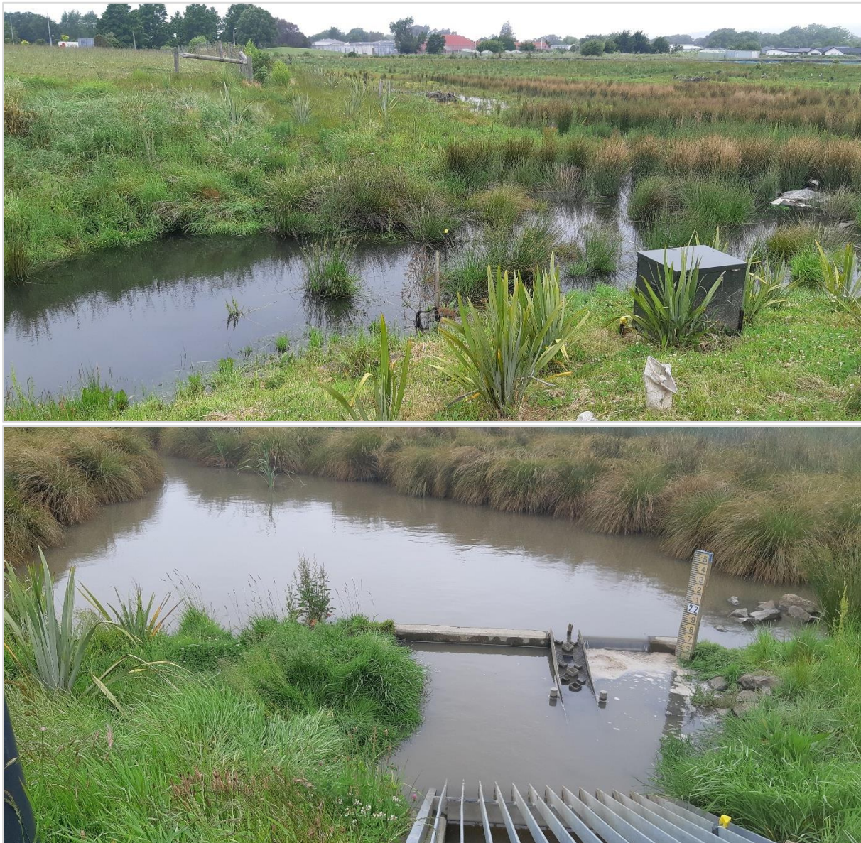
Figure 3-5: Curlett wetland inlet (top) and outlet (bottom). Photos taken 28 November 2021 (the day after Event 4). Note water is more turbid at the outlet than the inlet.
