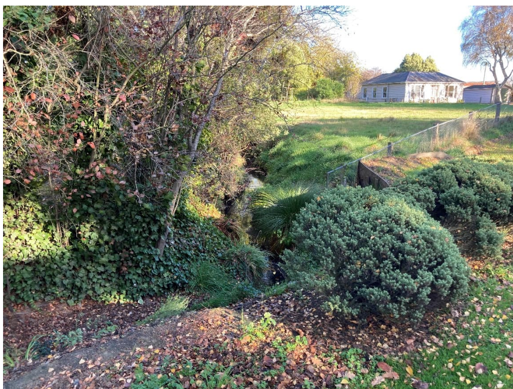
Plate 4. Nottingham Stream at Candys Road monitoring site (samples are taken from the culvert at the foreground of the photo)
