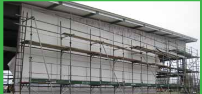
External view of Graham Condon Leisure Centre under construction © Copyright
