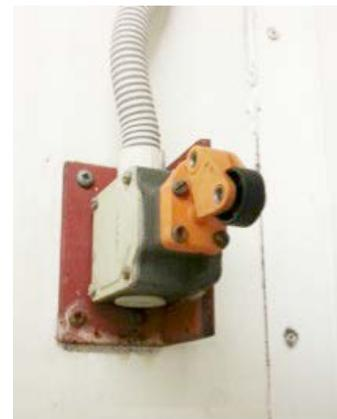
Repaired cooling room contact switch © Copyright
