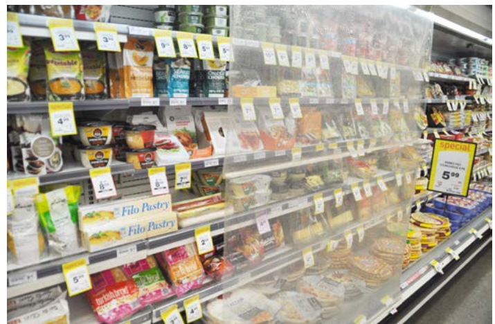
Repaired blinds on the vertical chillers © Copyright
