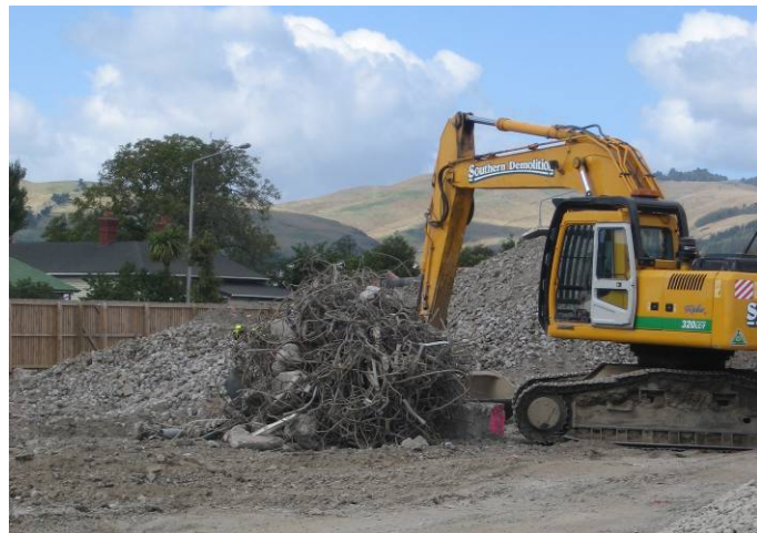
Re-bar being removed from the crushed concrete prior to crushing © Copyright
