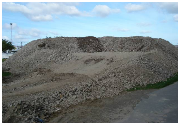
Concrete crushed for reuse on-site © Copyright
