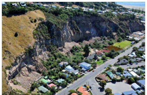
▲ Rock and debris falls on an approximately 50 m high cliff behind houses at the north end of Wakefield Avenue, Sumner.
