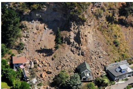
▲ Debris avalanche caused by cliff collapse (Raekura Place, Redcliffs) This landslide occurred in the main 22 February 2011 earthquake.
