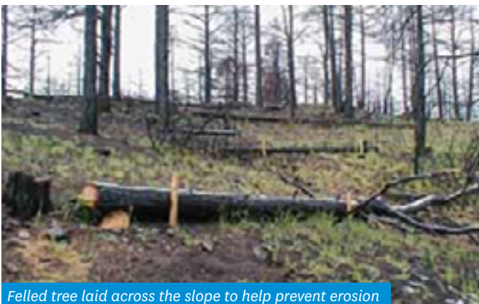
Felled tree laid across the slope to help prevent erosion
