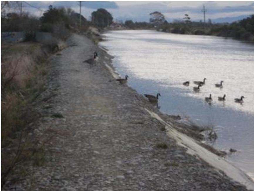
**Figure 1-13 Section 17 right bank – typical gravel fill stopbank**
