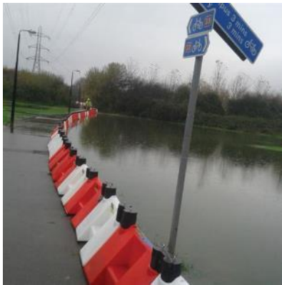
Temporary flood barrier (Image source: Fluvial Innovations, 2017).
