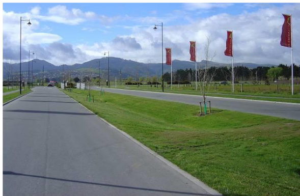
Swales collect and divert surface water to flow in desired location.
