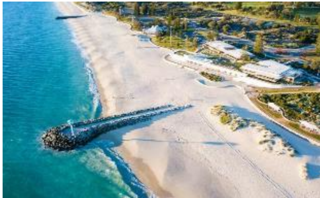
Concrete and rock groyne (Image source: Town of Cambridge, 2020).
