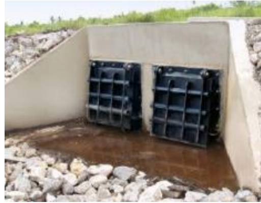
Flood gates allow water to flow out but not in prevent saltwater intrusion (Image source: Weida, 2018).
