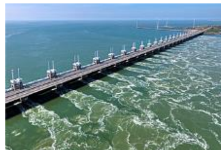
Permanent barrier in the Netherlands with gates that open and close (Image source: Dutch Water Sector, 2015).
