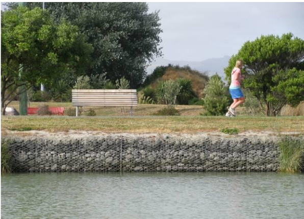
Seawall made of gabion baskets in Christchurch, New Zealand
