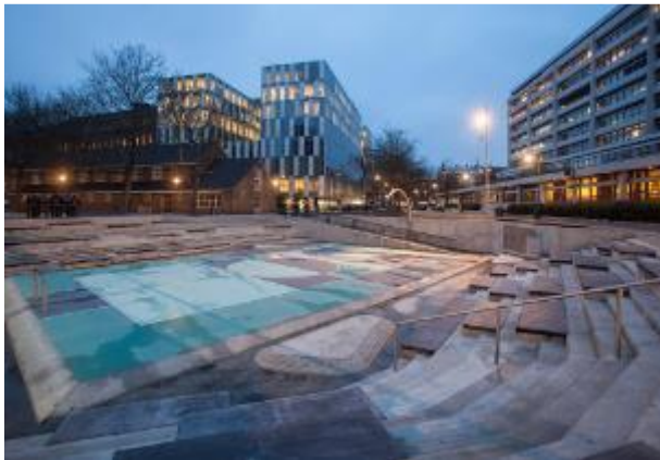
Water squares such as this in the Netherlands have a recreational purpose under dry conditions but can flood under wet conditions (Image source: Public Space, 2020).
