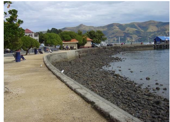
Concrete seawall in Akaroa, New Zealand with rocks in front of it.
