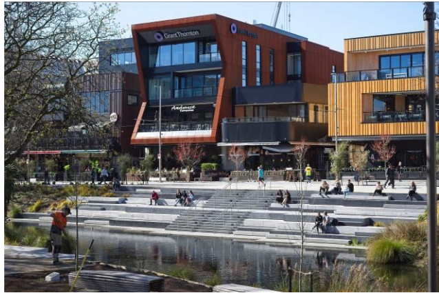
Concrete step revetment in Christchurch, New Zealand.
