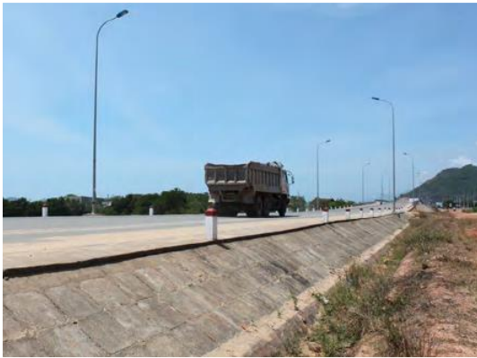
Raised road through a floodplain in Vietnam (Image source: Mallick et al., 2011).
