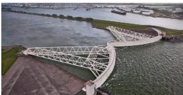
The wings of this movable barrier swing across the river as necessary in the Netherlands (Image source: Dutch Water Sector, 2018).
