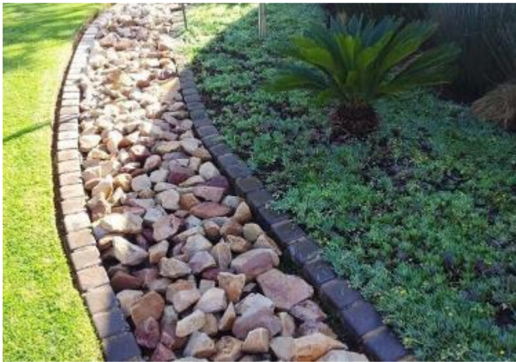
'French drain' utilises pipes below permeable materials (Image source: Tigard Sand and Gravel, 2020).
