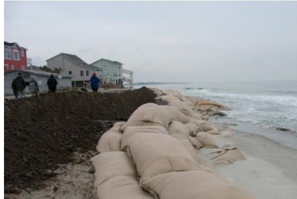
Emergency sand bagging (Image source: Coastal Care, 2010).
