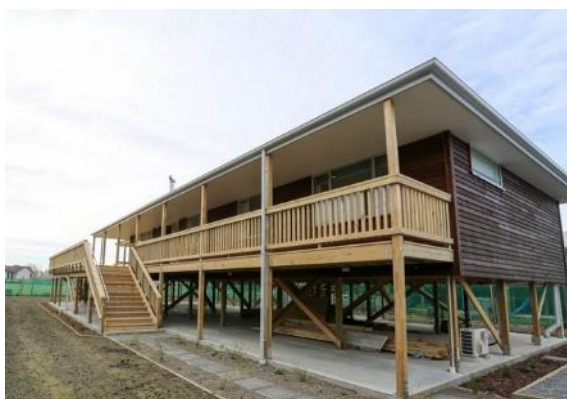
A house in Christchurch, New Zealand that is built to accommodate inundation (Image source: Property Value, 2021).
