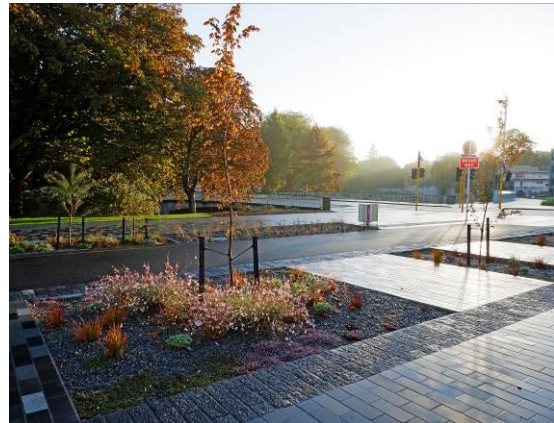
Rain gardens collect and filter storm water before it infiltrates into the groundwater.
