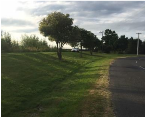
Vegetated stopbank protecting a road from flooding in Ngātea, New Zealand (Image source: Waikato Regional Council, 2019).
