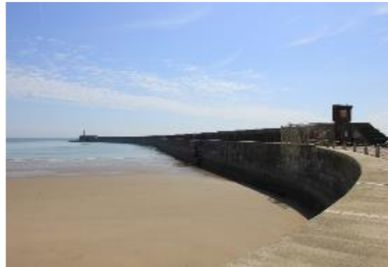
Concrete attached breakwater (Image source: The Coastal Path, 2013).
