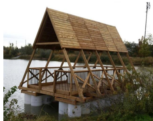
This amphibious pavilion is built on pontoons to increase its resilience to inundation (Image source: Buoyant Foundation Project, 2020).
