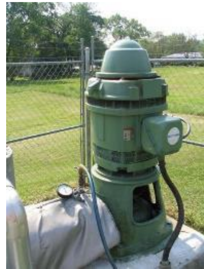
Groundwater well (Image source: United States Geological Survey, 2018).
