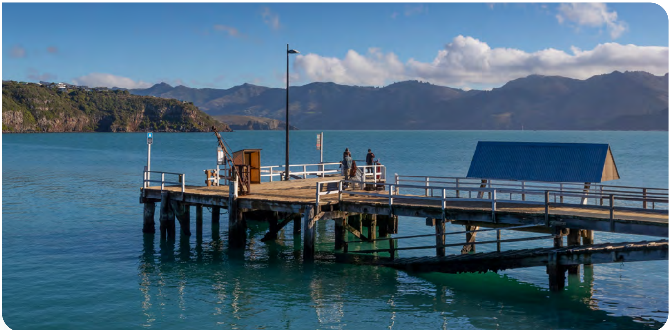
Diamond Harbour Wharf
