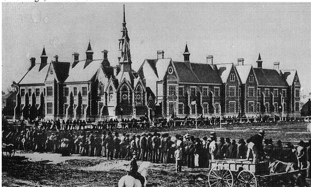
Figure 91. The Normal School, Cranmer Square, soon after its opening in April 1876. (The goalposts suggest that the crowd is watching a football match.) This became New Zealand's first teachers' training college in 1877. One of Christchurch's most important Gothic Revival buildings, it was converted to apartments in the early 1980s. E. R. Webb Collection, CM 5433
