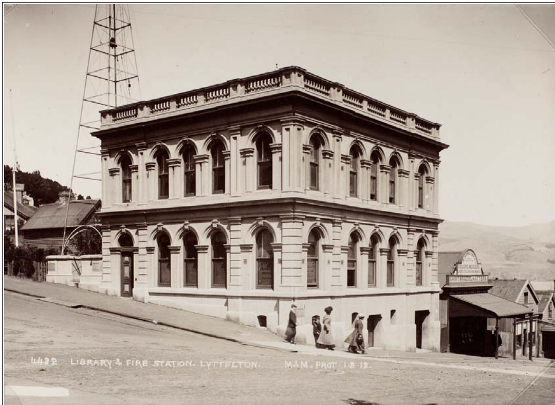
Figure 145. Library and fire station, Lyttelton, 1912. Source: Muir and Moodie photograph O.002051, MNZ
