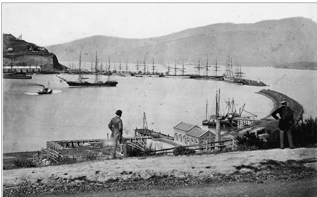
Figure 13. Part panorama of Lyttelton Harbour showing reclamation and breakwaters, 1882 Source: PA1-o-494-2, ATL
