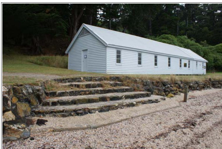
Figure 141. Restored single mens' quarantine barracks, Quail Island, 2014. Source: Ashley Mokena, DSC03535
