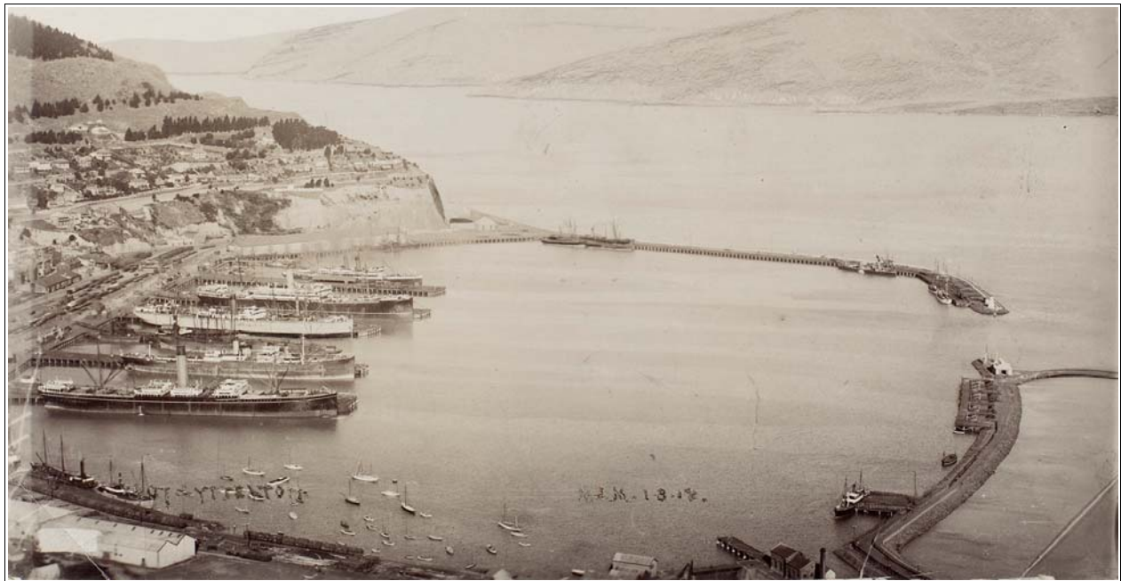
Figure 104. 1912 view of the port showing additional wharves associated with breakwaters and an increase in the number of warehouse buildings. Source: Muir and Moody photograph O.002047, MNZ
