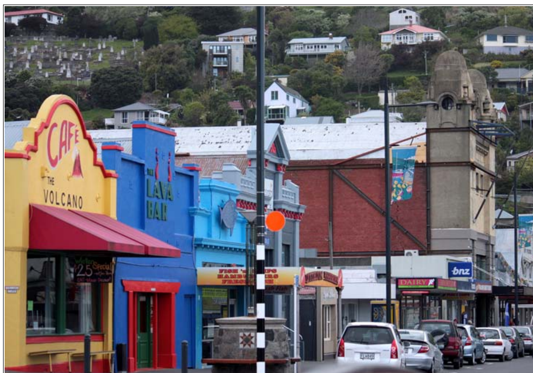
Figure 33. 2010 view of London Street, Lyttelton post September 2010 earthquake.
