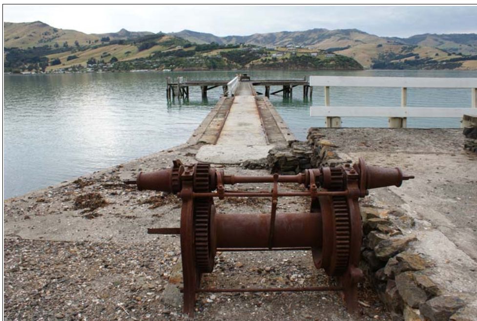
Figure 96. Duvauchelle wharf, 2014. Source: Ashley Mokena, DSC03300
