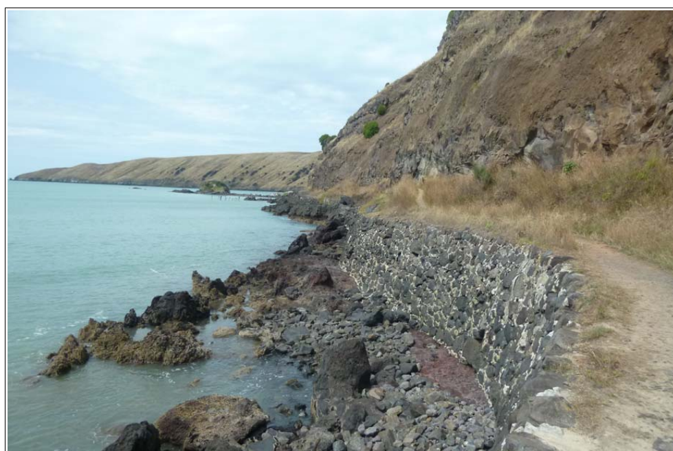
Figure 93. Okains Bay wharf road retaining wall, 2014. Source: Louise Beaumont, P1100036
