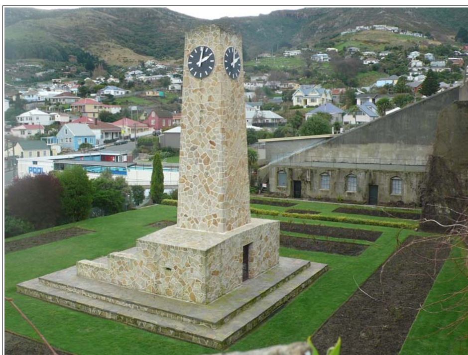
Figure 158. Upham Clock in the small reserve beside the gaol buildings, Lyttelton, 2010 Source: Louise Beaumont, P1110078
