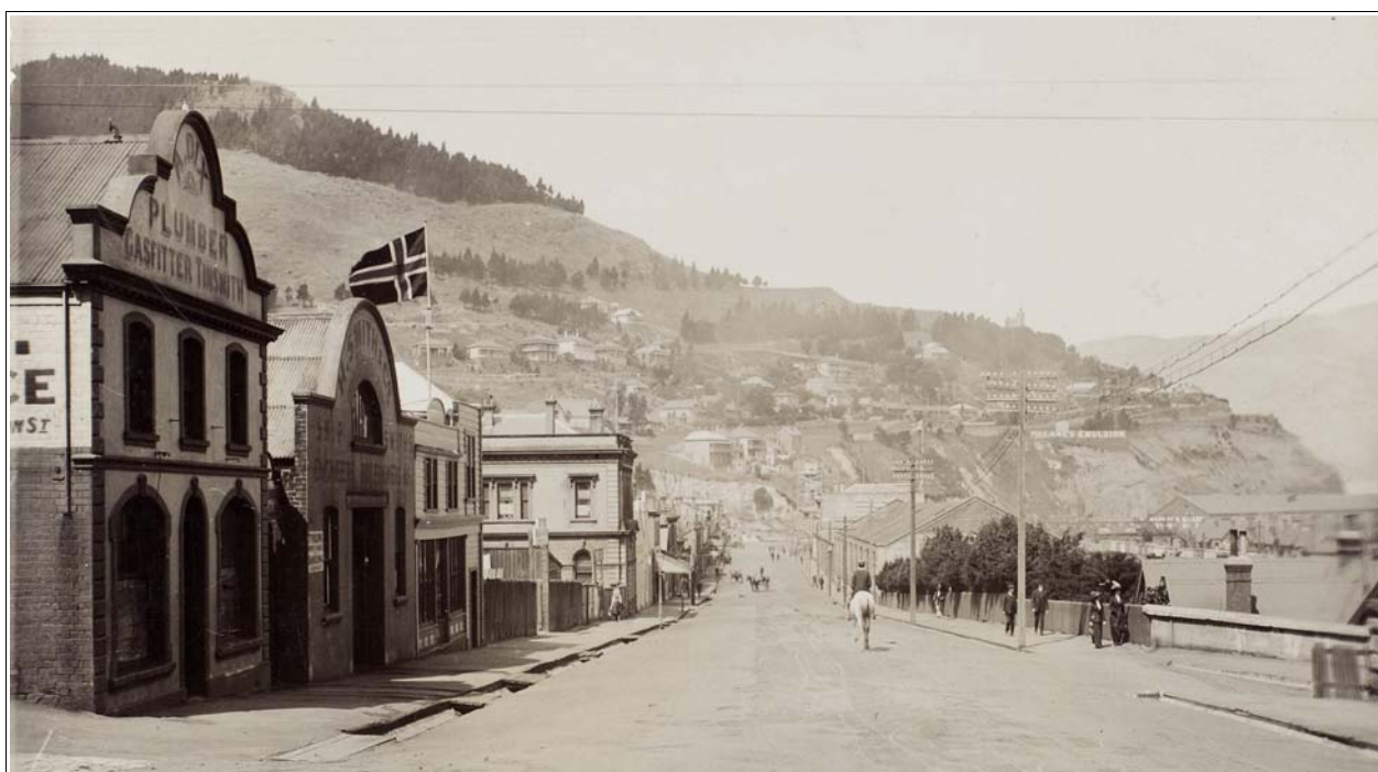
Figure 83. The business premises of A. Dix, Plumber, Gasfitter and Tinsmith and H. Smith & Co. Ships Engineers, Norwich Quay, Lyttelton, 1912. Source: Muir and Moody, O.002050, MNZ
