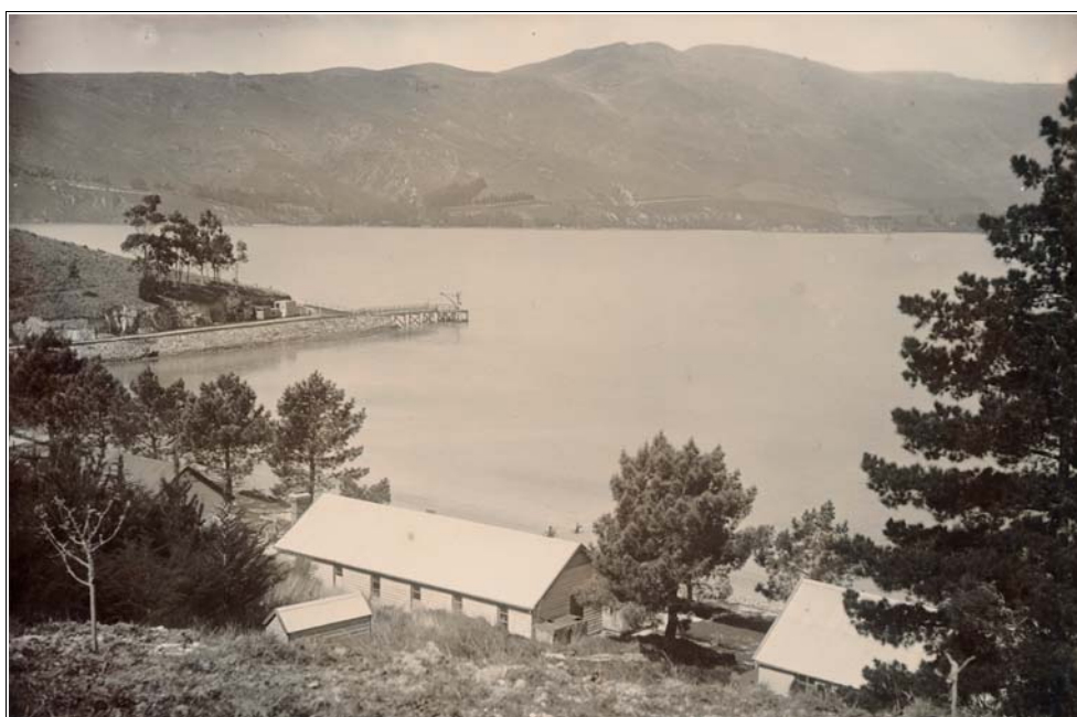
Figure 140. Quail Island quarantine buildings, early twentieth century. The mens' single barracks is centre mid-ground. Source: PA7-53-19, ATL
