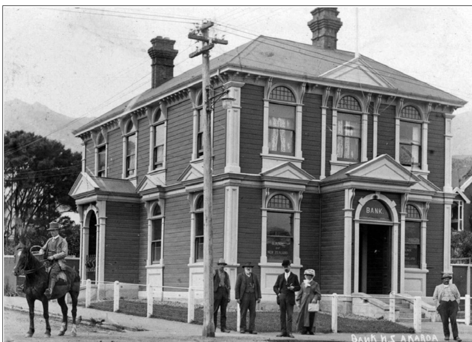
Figure 29. Bank of New Zealand, 1912. Source: Shuttleworth collection
