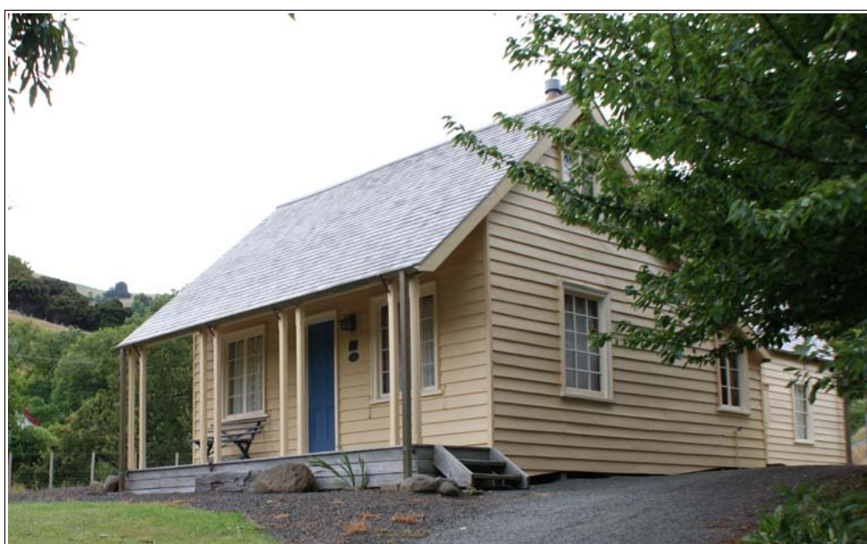
Figure 21. Restored Pavitt cottage, Robinsons Bay, 2014. Source: Ashley Mokena, DSC03273
