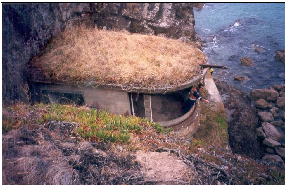
Figure 121. Battery Point, Number 1 searchlight shelter. Source: Phil Moore, 2008
