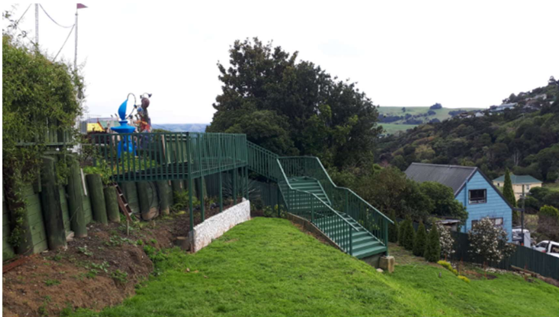
Figure 10: The stair structure linking the upper floor of the Café Building and Linton, with the 74 Rue Balguerie, the new area of garden.
