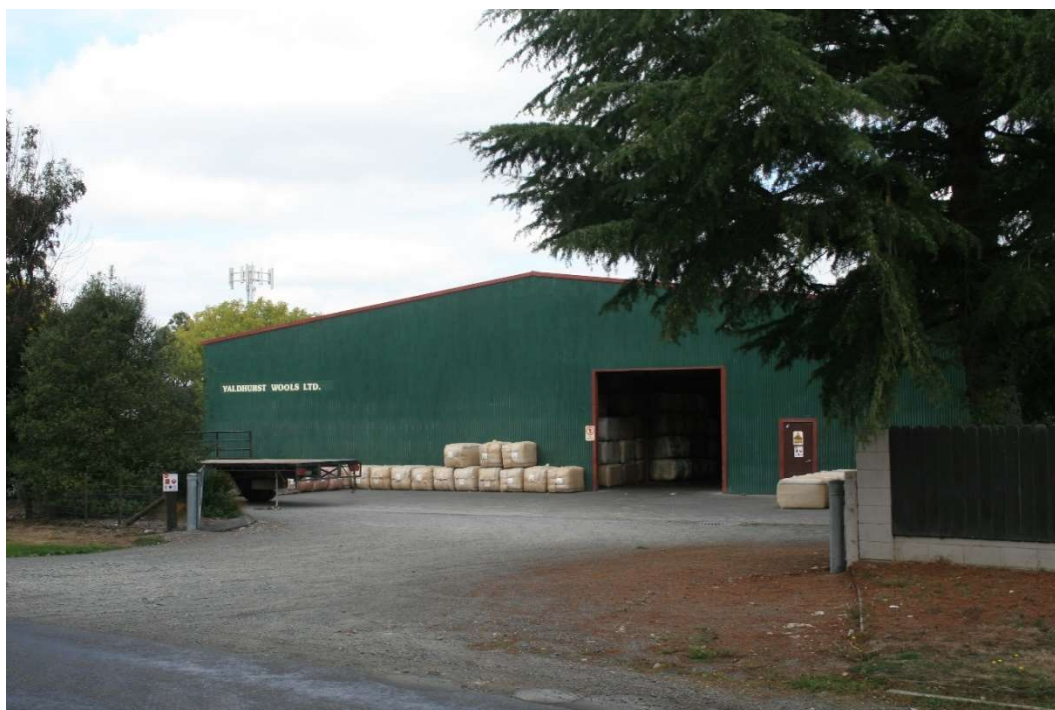
Figure 2 Yaldhurst Wools Ltd at 30 School Road, viewed from School Road. This building has a footprint of approximately 1,300 m 2 . Note the simple built form with pitched roof, minimal glazed area, set amongst / buffered by vegetation, supporting rural landuse activity. Photograph by J. Head, 30 March 2021.
