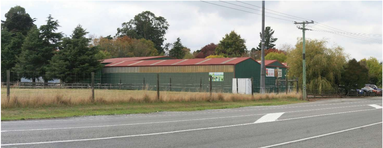
Figure 3. Yaldhurst Wools Ltd. at 30 School Road located at eastern end of site viewed from SH73. Photograph by J. Head, 30 March 2021.
