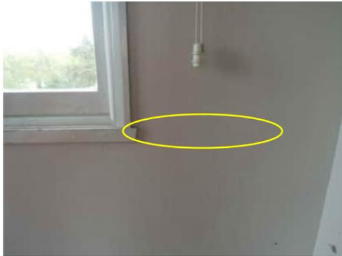
3.17 | HORIZONTAL HAIRLINE CRACK IN GRID D COLUMN AT BOTTOM OF WINDOW
