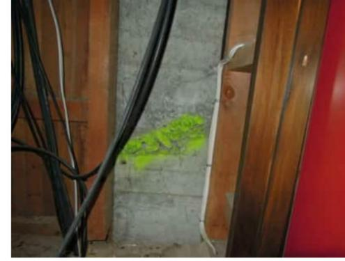
**3.52** POOR QUALITY CONCRETE BETWEEN TWO VOIDS
