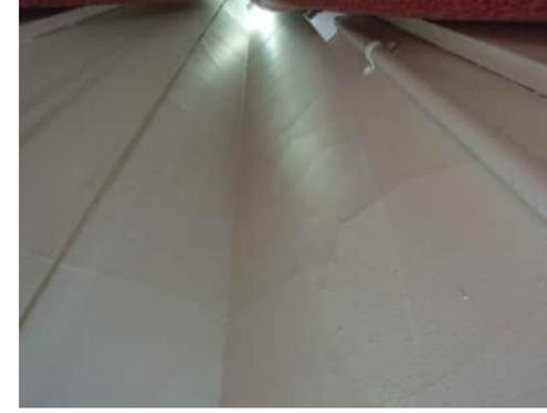
2.32 | CRAZED CRACKS UP WHOLE HEIGHT OF COLUMN AT GRID 21
