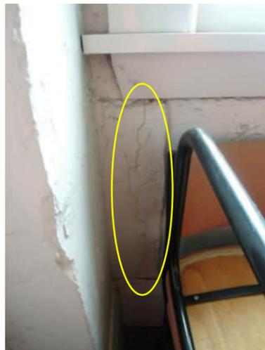
1.9 0.9MM VERTICAL CRACK FROM BOTTOM OF WINDOW IN GRID C COLUMN
