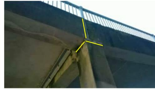
**R27** | CRACK SHOWN IN PHOTO R26 CONTINUES THROUGH BEAM TO TOP OF COLUMN. VERTICAL CRACK THROUGH BEAM WHERE RAMP AND LANDING INTERSECT
