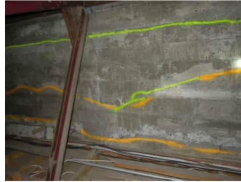
**3.50** UPPER CRACK IS THROUGH POUR LINE. POOR QUALITY CONCRETE AT BOTTOM. MIDDLE HORIZONTAL CRACK 0.8 TO 1.6mm WIDE
