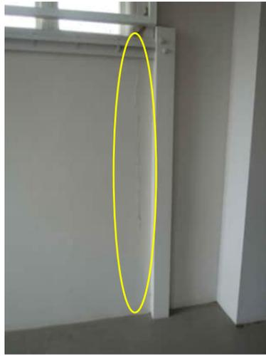
2.13 | VERTICAL CRACK BETWEEN GRID D COLUMN AND WALL
