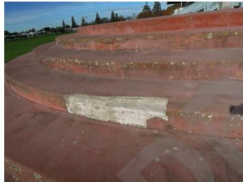
**EXT.5** | SPALLING DAMAGE TO TOP OF STEP
