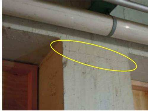
**0.36** TYPICAL CRACK NEAR TOP OF COLUMN, ON ALL FACES OF COLUMN
