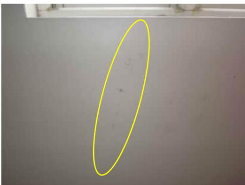
2.33 | HAIRLINE DIAGONAL CRACK BELOW WINDOW BETWEEN GRID 9 AND 10 WITH SOME MOISTURE SEEPAGE
