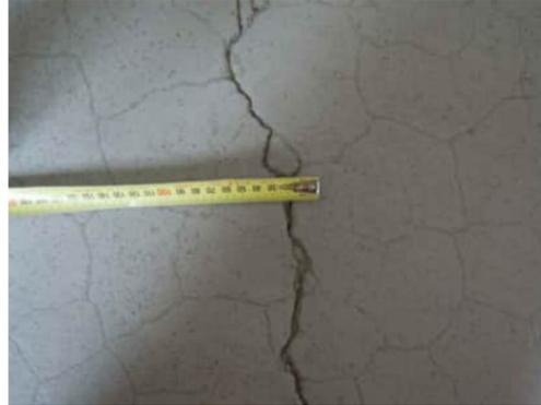
2.3 | CRACK RUNNING DIAGONALLY ACROSS SLAB, UP TO 10MM
