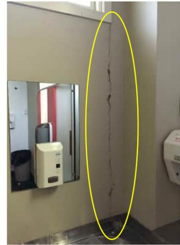
1.15 | CRACK BETWEEN GRID D COLUMN AND WALL 2-3MM WIDE WITH SPALLING UP TO 25MM ON SURFACE
