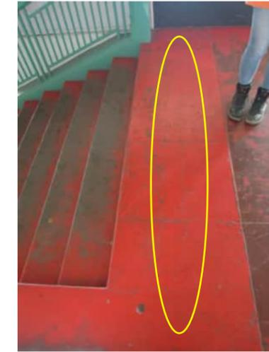
3.8 | CRACK IN COATING ALONG TOP OF STAIRS SPALLING UP TO 10MM WIDE AT SURFACE
