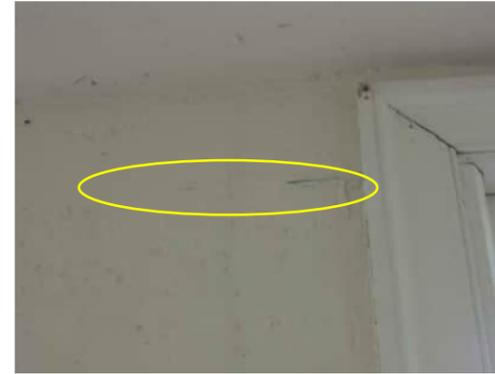
2.8 | CRACK NEAR TOP OF WINDOW ON COLUMN BETWEEN GRID C AND GRID D
