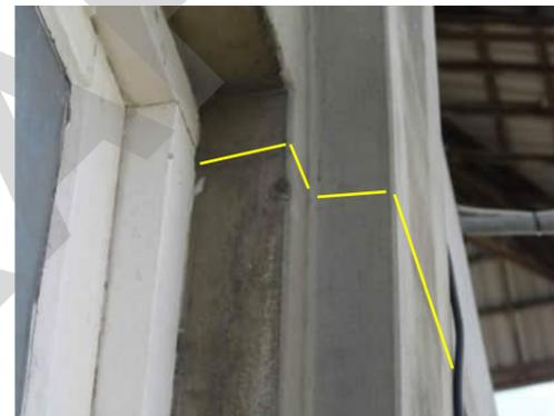
**EE19** | HORIZONTAL CRACK IN COLUMN BETWEEN GRID B AND C
