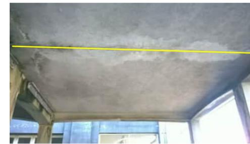
**R28** | CRACK ON UNDERSIDE OF LANDING SLAB
