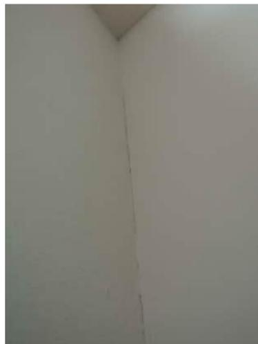
**3.33** | SEPARATION BETWEEN COLUMN AND SERVICE SHAFT AT GRID 13
