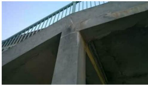
**R29** | CRACKS TO BEAM AND COLUMN
