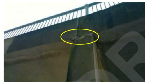
**R30** | CRACK BETWEEN BEAM AND COLUMN
