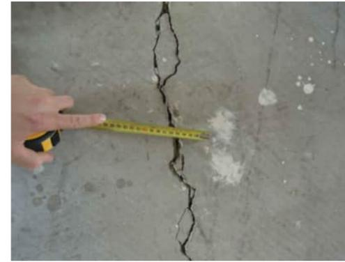
1.4 SPALLING OF CRACK BETWEEN GRID C COLUMNS
