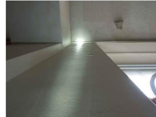
**0.51** SIGN OF MOISTURE DAMAGE TO TOP OF COLUMN ON GRID 17, ALSO OCCURS AT GRID 20
