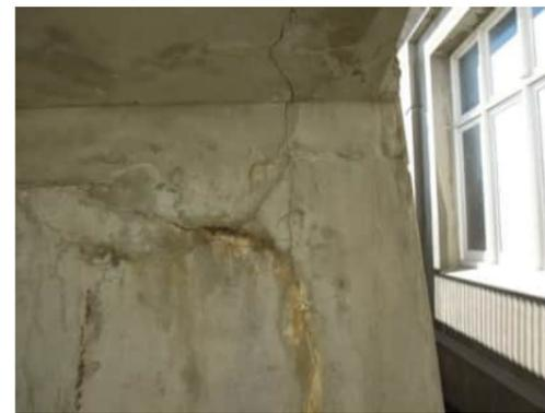
**S14** | VERTICAL CRACKS UP TO 0.8MM WIDE ON THE UNDERSIDE OF THE STAIRS AND DOWN THE WALL BELOW THE STAIRS
