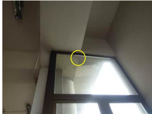
3.39 | CRACK ON UNDERSIDE OF BEAMS BETWEEN GRID E BEAM AND BEAM FOR THE LIFT SHAFT EXTENSION, NEAR GRID 11
