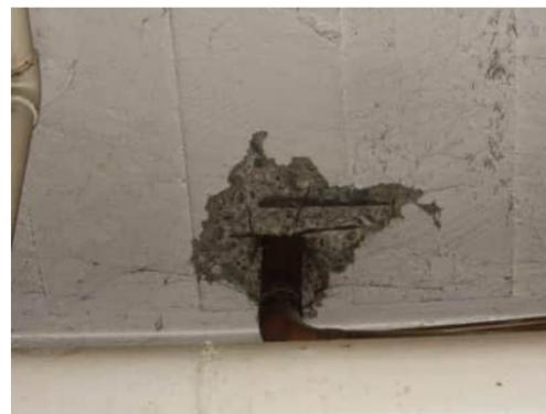
**0.61** PIPE THROUGH CEILING WITH SPALLING WHICH HAS EXPOSED REINFORCING
