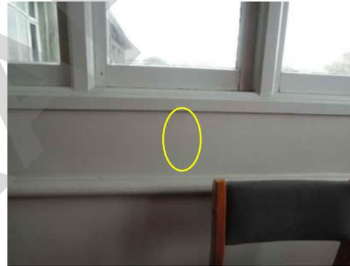
3.19 | HAIRLINE CRACK IN WALL BELOW WINDOW BETWEEN GRID D AND E
