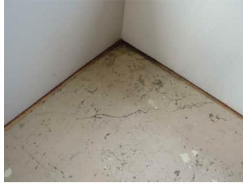
3.14 | CRACKS IN CORNER UP TO 0.6MM
