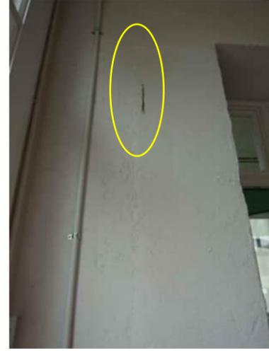
1.26 | DAMAGE TO SURFACE BETWEEN GRID 1 COLUMN AND CONCRETE DOOR FRAME
