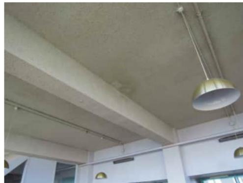
3.47 | MOISTURE DAMAGE TO BEAM AND CEILING AT GRID 15
