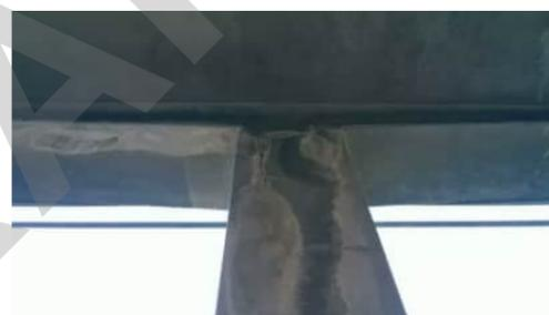
**R31** | SIGNIFICANT VERTICAL CRACK NEAR TOP OF COLUMN
