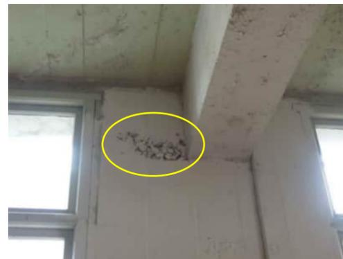
**0.45** POORLY COMPACTED CONCRETE AT TOP OF COLUMN, TYPICAL BETWEEN GRID 1 AND GRID 4
