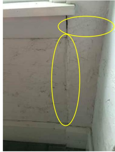
1.25 | CRACK IN CORNER OF GRID C COLUMN BELOW WINDOW
