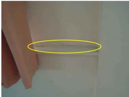
**0.52** HORIZONTAL CRACK IN WALL ON GRID 17 IN LINE WITH BOTTOM OF WINDOW
