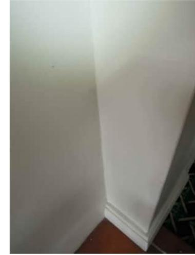
**0.39** SEPARATION BETWEEN GRID 13 COLUMN AND GIB LINED WALL
