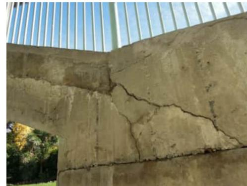
**S18** | CRACKS UP TO 15MM AT TOP OF WALL WHERE STAIRS BEGIN
