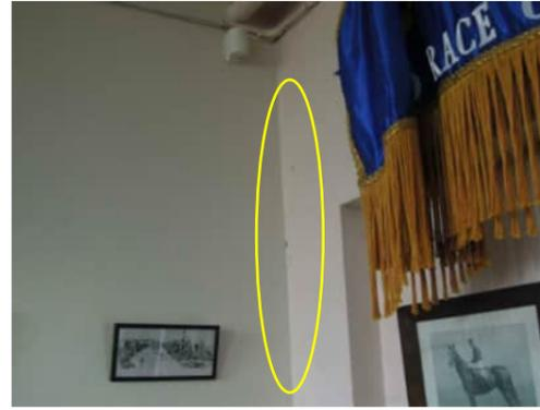
2.15 | SEPARATION BETWEEN GRID D COLUMN AND WALL
