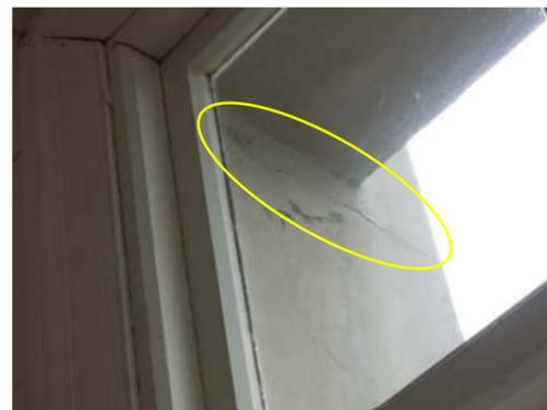
2.9 | CRACK NEAR TOP OF WINDOW ON COLUMN BETWEEN GRID C AND GRID D CONTINUES TO EXTERIOR
