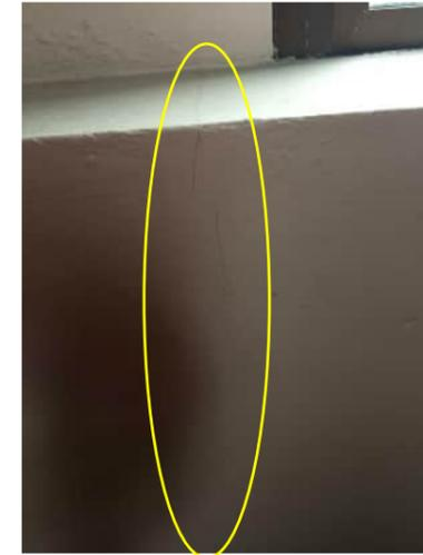
1.28 | VERTICAL CRACK UP TO 0.2mm BELOW WINDOW AT GRID 11 IN LIFT SHAFT EXTENSION
