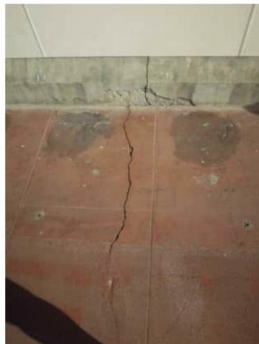
**EXT.8** | CRACK IN SLAB AND RETAINING WALL
