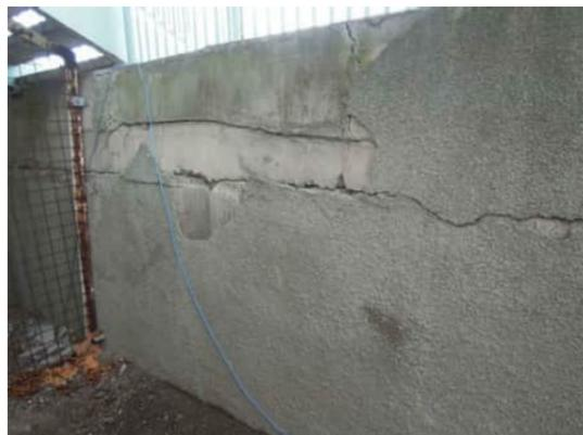
**RW.5** SIGNIFICANT CRACKS UP TO 10MM AND DAMAGE TO RENDER
