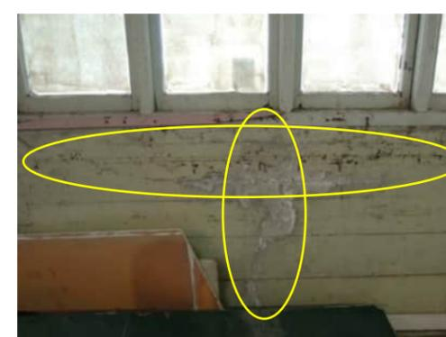
**0.46** HORIZONTAL AND VERTICAL CRACK BELOW WINDOW BETWEEN GRID 4 AND 5
