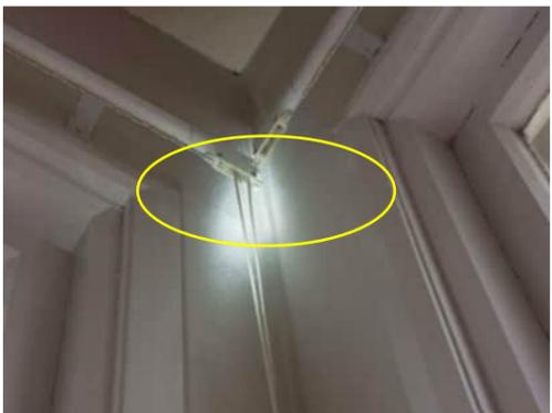
3.21 | HAIRLINE CRACK NEAR TOP OF WINDOW IN GRID E COLUMN
