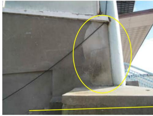
**EE13** | CRACKING TO WALL ABOVE GRID A COLUMN
