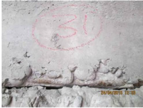
**RW.13** | SIGNIFICANT HORIZONTAL CRACK AT JOINT AND EXPOSED REINFORCEMENT AT APPROXIMATELY 600MM FROM THE TOP OF THE WALL
