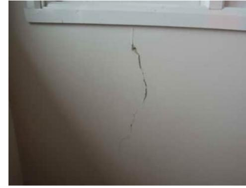
3.16 | 3MM VERTICAL CRACK BELOW WINDOW, CRACK HAS SPALLED UP TO 15MM
