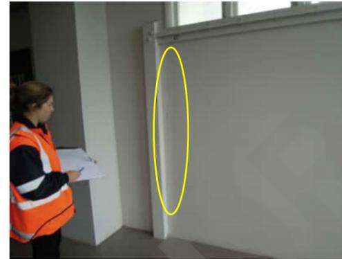
2.18 | 0.7MM VERTICAL CRACK BETWEEN GRID D COLUMN AND
