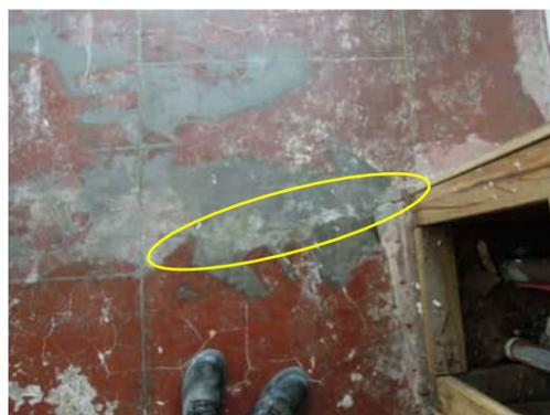
3.9 | CRACK UP TO 5MM WHICH HAS PREVIOUSLY BEEN PARTIALLY REPAIRED
