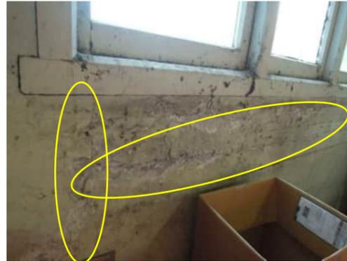
**0.49** HORIZONTAL AND VERTICAL CRACK BELOW WINDOW BETWEEN GRID 7 AND 8
