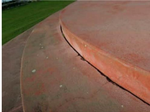
**EXT.4** | SEPARATION BETWEEN SLAB AND FIRST STEP UP TO 25MM
