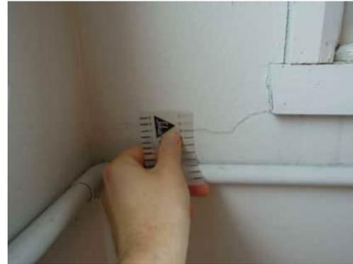
3.38 | 0.3MM HORIZONTAL CRACK IN GRID 21 COLUMN FROM CORNER OF WINDOW
