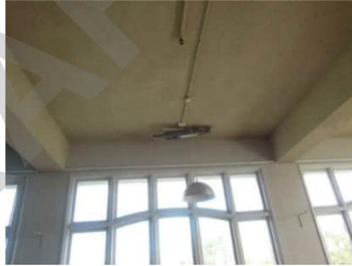
3.43 | HEATER INADEQUATELY CONNECTED TO CEILING - HAZARD
