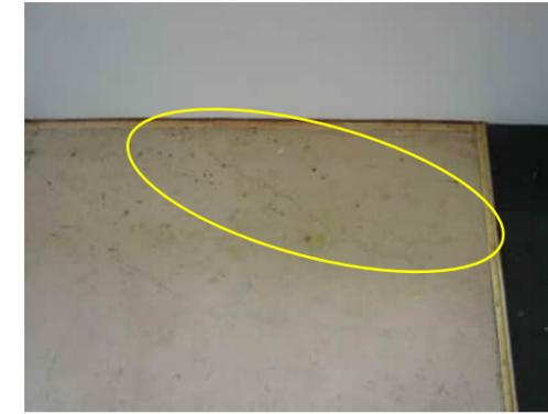
3.4 | DIAGONAL CRACK IN CORNER UP TO 1.2MM
