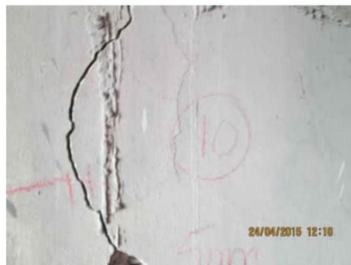
**RW.10** 1.8M LONG VERTICAL CRACK, UP TO 5MM WIDE, STARTING FROM THE BOTTOM OF THE WALL
