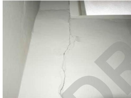
1.18 | 1.6MM VERTICAL CRACK BETWEEN WALL AND COLUMN AT GRID D
