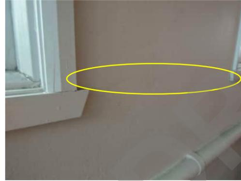
3.42 | HORIZONTAL HAIRLINE CRACK ON GRID 12 COLUMN AT BOTTOM OF WINDOW
