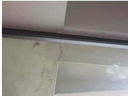
3.41 | CRACK ON UNDERSIDE OF BEAMS BETWEEN GRID E BEAM AND BEAM FOR THE LIFT SHAFT EXTENSION, NEAR GRID 11
