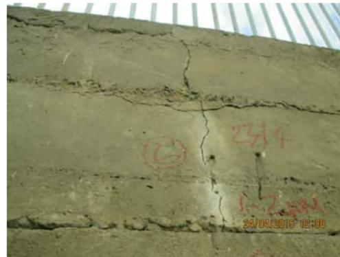
**RW.8** VERTICAL CRACK FROM TOP OF WALL TO JOINT AND A HORIZONTAL CRACK RUNNING THROUGH
