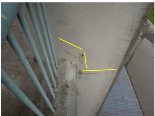
**EW21** | CRACKING TO GRID E COLUMN NEAR WHERE STAIRS CONNECT AT SECOND FLOOR UP TO 0.5MM
