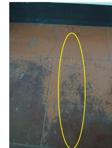
3.12 | CRACK IN COATING UP TO 3MM WIDE
