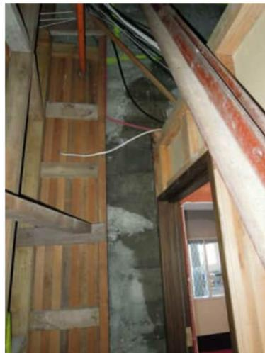
**3.53** WATER INGRESS DAMAGE AT GRID 13 THROUGH CRACKING AT TOP
