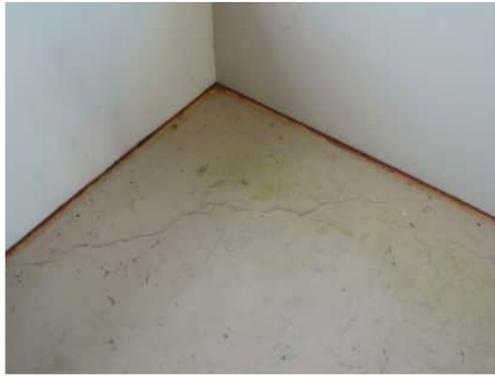
3.1 | DIAGONAL CRACKS AT CORNER OF BUILDING UP TO 3MM
