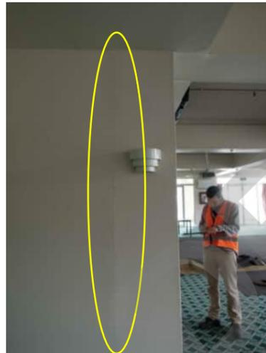
**0.41** SEPARATION TO GIB LINING BETWEEN GRID 17 COLUMN AND WALL
