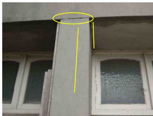
**EW22** | VERTICAL CRACKING TO CENTRAL COLUMN AND SEPARATION BETWEEN THE COLUMN AND THE WALL BETWEEN THE SECOND AND THE THIRD FLOOR
