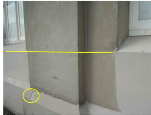
**EW3** | 0.2MM HORIZONTAL CRACK NEAR BASE OF CENTRAL COLUMN
