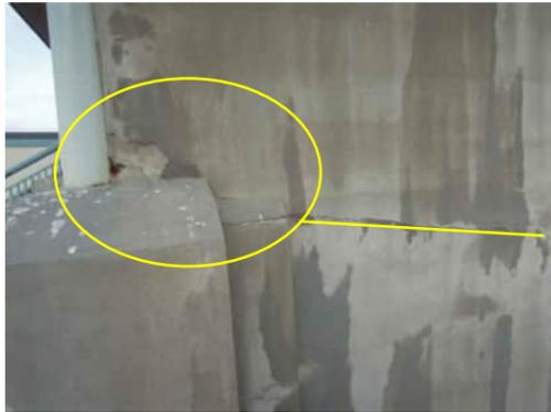
**EW17** | HORIZONTAL CRACK AT GRID A COLUMN WITH SPALLING AND EVIDENCE OF RUST
