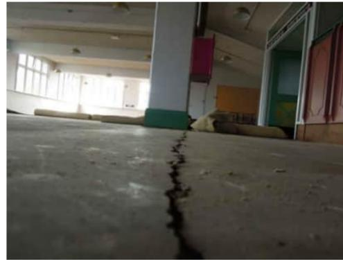
1.3 CRACK BETWEEN GRID C COLUMNS UP TO 10MM WIDE WITH 5MM VERTICAL DISPLACEMENT
