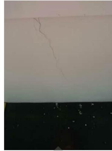
3.15 | VERTICAL CRACK BELOW WINDOW UP TO 0.4MM NEAR GRID C
