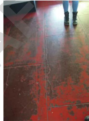
3.7 | CRACK IN COATING, SPALLING UP TO 10MM WIDE AT SURFACE
