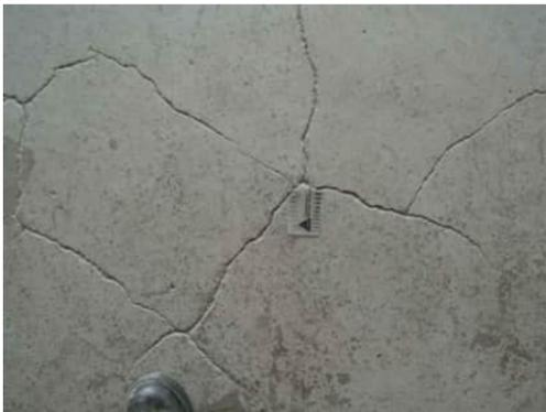
2.5 | CRACKING TO SLAB UP TO 5MM
