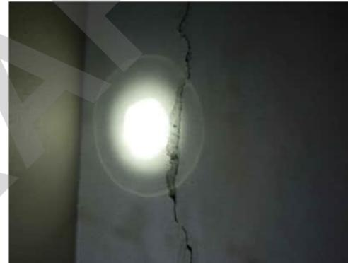
1.19 | SPALLING OF CRACK BETWEEN WALL AND COLUMN AT GRID D
