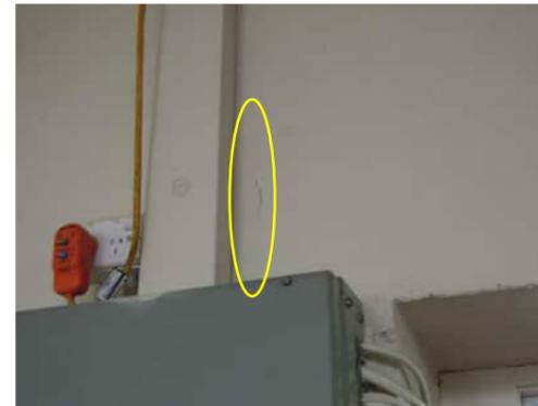
2.23 | VERTICAL CRACK IN BEAM ABOVE GRID 5 COLUMN
