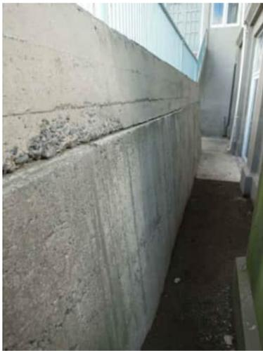
**RW.1** VIEW OF RETURN OF RETAINING WALL AT EASTERN END, JOINT IS UP TO 10MM
