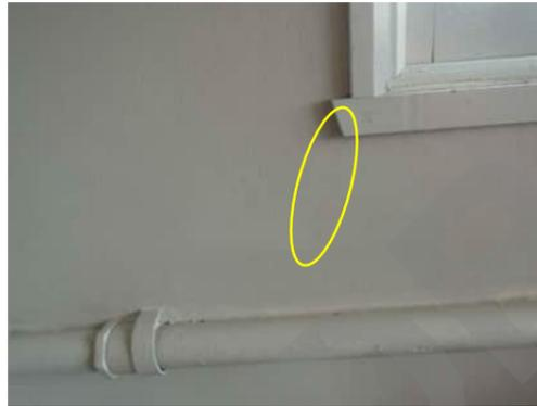
3.18 | HAIRLINE CRACK FROM CORNER OF WINDOW IN GRID D COLUMN
