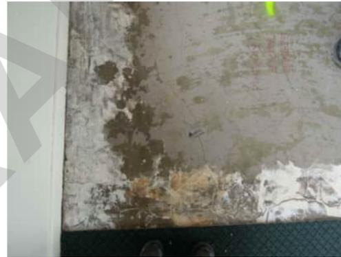
2.7 | PARTIALLY FILLED CRACKS ON SLAB, UP TO 0.8MM
