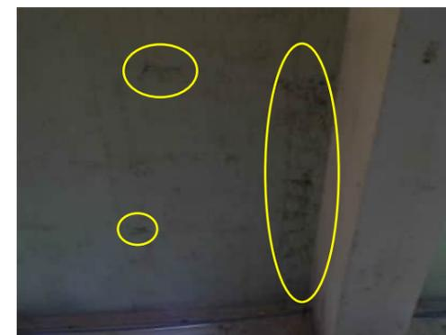
**0.59** EXPOSED SLAB BOTTOM REINFORCEMENT, IN THE BAY BETWEEN GRID 8 AND GRID 9
