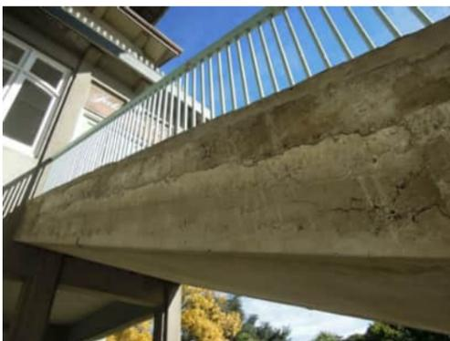
**S19** | CRACKS ALONG STRINGER AS WELL AS POORLY COMPACTED CONCRETE
