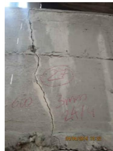
**RW.12** APPROXIMATELY 600MM LONG VERTICAL CRACK, STARTING FROM THE TOP OF THE WALL, UP TO 3MM WIDE
