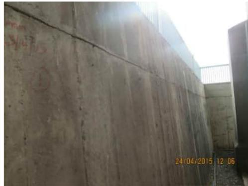
**RW.2** VIEW OF RETURN OF RETAINING WALL AT WESTERN END, JOINT IS 0.6MM
