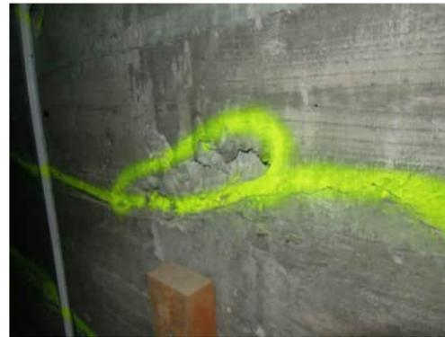
**3.51** POOR QUALITY CONCRETE ON GRID 4 WITH 2MM WIDE HORIZONTAL CRACK
