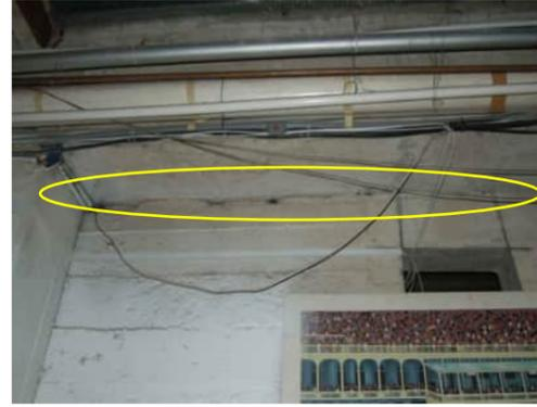
**0.38** SEPARATION BETWEEN CONCRETE WALL AND BEAM/COLUMNS BETWEEN GRID 12 AND 13
