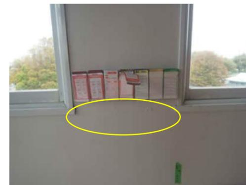
**3.36** | EVIDENCE OF MOISTURE ON GRID 20 COLUMN. SIMILAR AT GRID 3 AND 5
