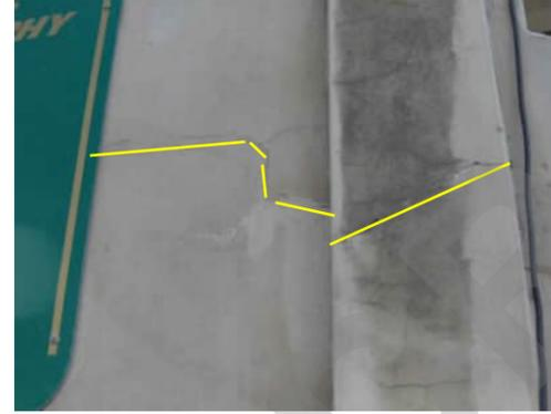
**EE18** | HORIZONTAL CRACK IN WALL AND COLUMN BETWEEN GRID B AND C
