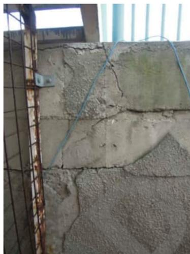
**RW.6** SIGNIFICANT CRACKS BELOW STAIRS UP TO 3MM
