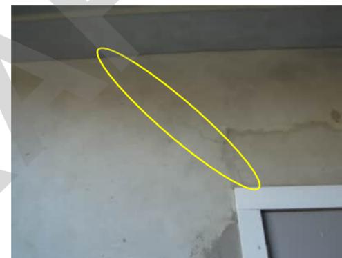
**0.66** DIAGONAL CRACK ON EXTERIOR FACE OF CONCRETE WALL
