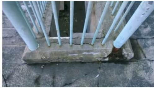
**R25** | CRACKING TO THE BEAM AND LANDING SLAB BETWEEN THE STAIRS AND RAMP, CONCRETE BROKEN OUT AROUND HANDRAIL
