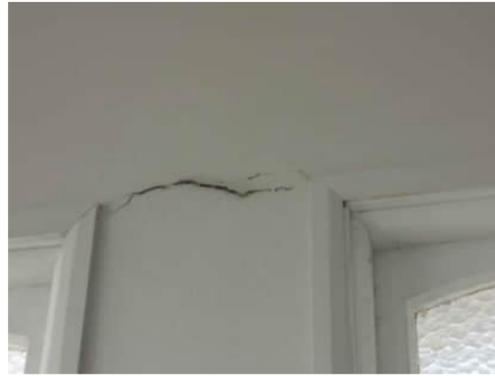
2.14 | SIGNIFICANT HORIZONTAL CRACK WITH SPALLING ON WALL
