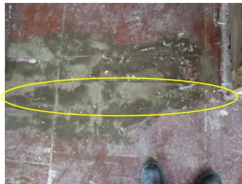
3.10 | CRACK UP TO 2MM WHICH HAS BEEN PREVIOUSLY REPAIRED
