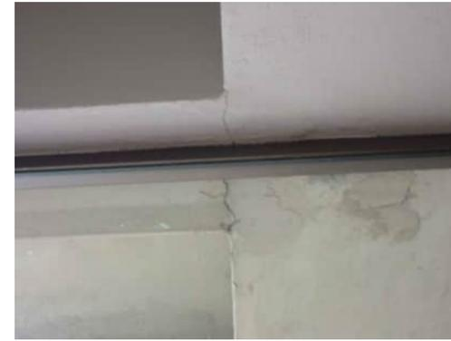
3.40 | CRACK ON UNDERSIDE OF BEAMS BETWEEN GRID E BEAM AND BEAM FOR THE LIFT SHAFT EXTENSION, NEAR GRID 10
