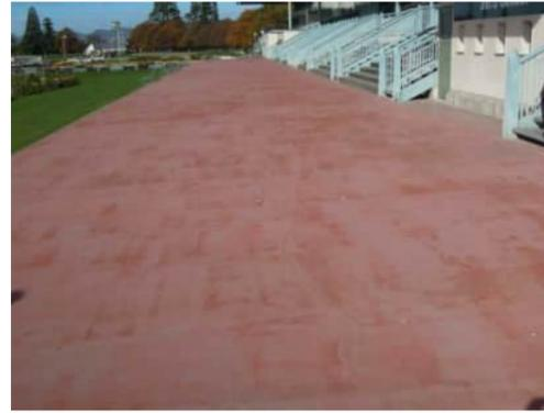
**EXT.1** | CRACK ALONG ENTIRE LENGTH OF SLAB
