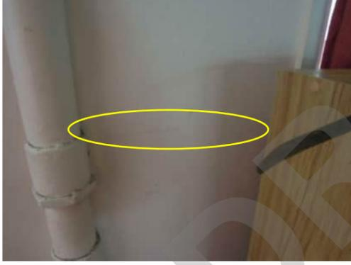
2.30 | HORIZONTAL HAIRLINE CRACK IN COLUMN AT GRID 14 (GRID 8, 17 AND 19 SIMILAR)
