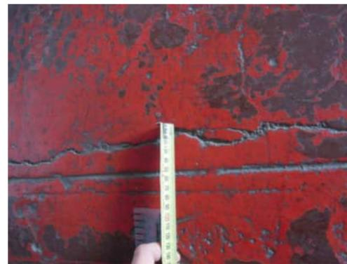
3.11 | CRACK IN COATING SPALLING UP TO 10MM WIDE AT SURFACE
