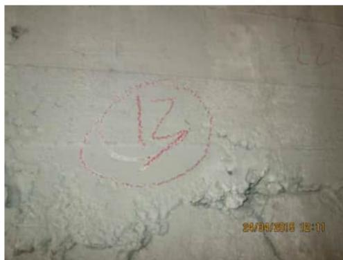
**RW.11** SEVERE CONCRETE SPALLING
