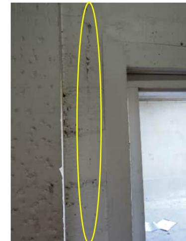
**0.67** VERTICAL FULL HEIGHT CRACK IN CONCRETE WALL PANEL ON INTERIOR FACE
