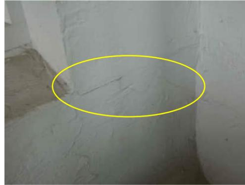
1.14 | CRACK FROM BOTTOM CORNER OF WINDOW IN GRID C COLUMN
