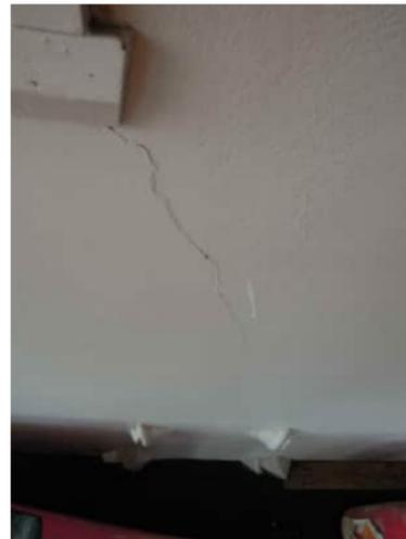
3.22 | 0.3MM DIAGONAL CRACK FROM BOTTOM OF WINDOW AT GRID 2 COLUMN
