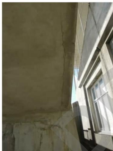
**S16** | CRACK ON UNDERSIDE OF STAIRS UP TO 4MM WIDE
