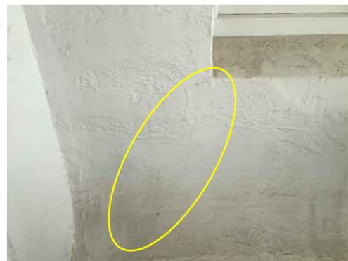
1.22 | DIAGONAL CRACK FROM BOTTOM CORNER OF WINDOW IN GRID C COLUMN
