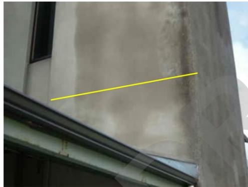
**EW18** | CRACK IN LIFT SHAFT NEAR FLOOR LEVEL OF FIRST FLOOR
