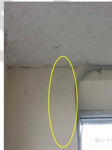
**0.54** CRACKS AT TOP OF GRID 21 COLUMN
