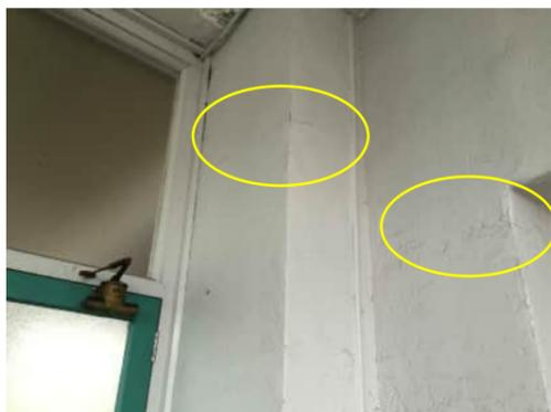
1.21 | HORIZONTAL CRACK IN GRID C COLUMN 0.5m FROM TOP OF COLUMN. CRACK IN WALL NEAR TOP OF WINDOW FRAME
