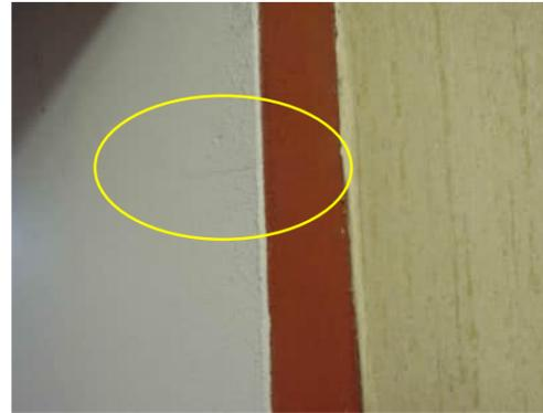
3.23 | HAIRLINE HORIZONTAL CRACK 2M UP THE GRID 9 COLUMN
