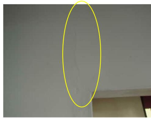
**3.27** | VERTICAL CRACK IN SHEAR WALL ABOVE DOOR OPENING NEAR GRID 12
