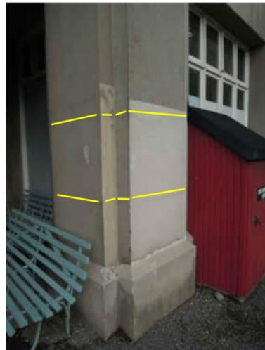
**EW5** | 0.2MM HORIZONTAL CRACKS NEAR BASE OF GRID C COLUMN
