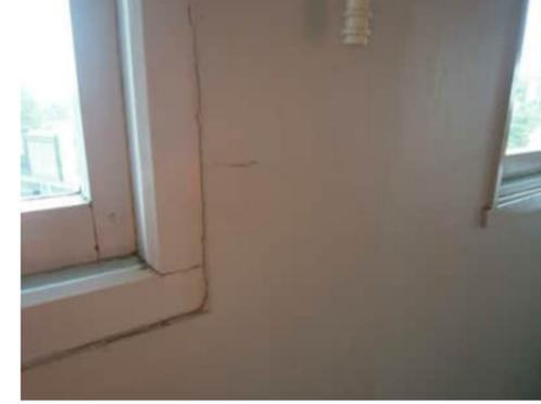
**3.32** | SEPARATION OF GIB FROM WINDOW FRAME AND HORIZONTAL CRACK UP TO 0.8MM IN GRID 6 COLUMN
