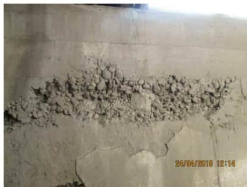
**RW.3** TYPICAL AREA WITH POORLY COMPACTED CONCRETE
