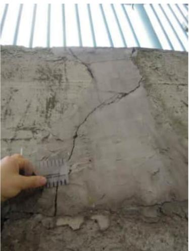
**RW.9** CRACKS UP TO 2.5MM WHICH HAVE PREVIOUSLY BEEN REPAIRED BUT HAVE REAPPEARED
