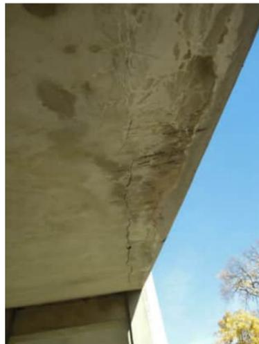
**S15** | CRACK ON UNDERSIDE OF STAIRS UP TO 4MM WIDE
