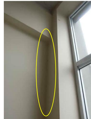
**0.43** SEPARATION BETWEEN GRID 21 COLUMN AND WALL
