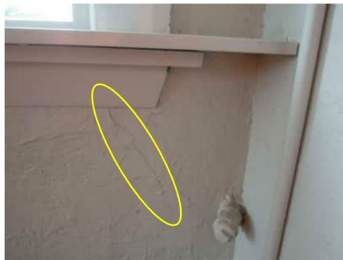
1.11 0.3MM DIAGONAL CRACK FROM BOTTOM OF WINDOW IN GRID C COLUMN
