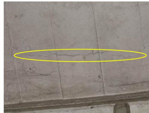
**0.62** SIGNIFICANT CRACKS IN THE CEILING NEAR GRID 12/D
