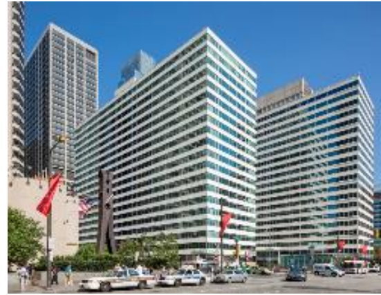
Figure 6: Buildings with a blunt roof form.
