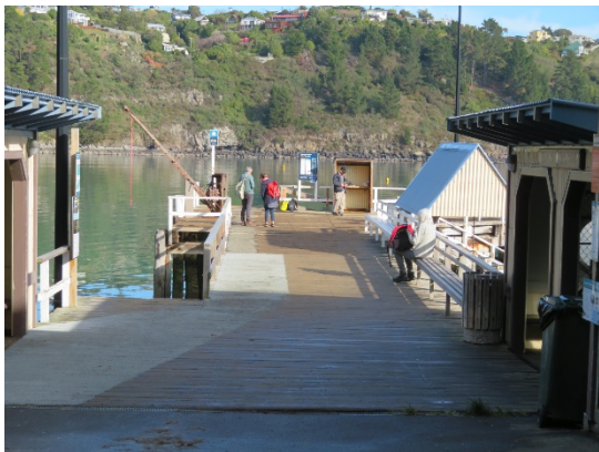
Source: T Ussher June 2020 The wharf seen from the carpark with the shelters either side. The 1916 shelters were replaced in 2008.
