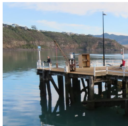
Source: T. Ussher 2020 The current smaller crane mounted on the edge, and not towards centre of the wharf enabling it to reach around three sides.
