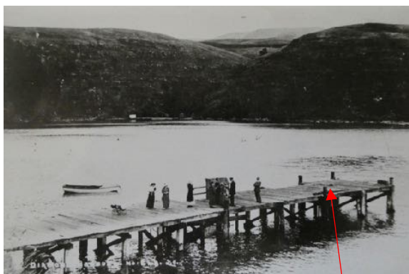
Source: Stoddart Album, DHHS. Photo c1913. The 1874 jetty without the crane. The crane was located in the centre of the end bay of the jetty as arrowed. Is the dark spot in the photo evidence of the removed crane?
