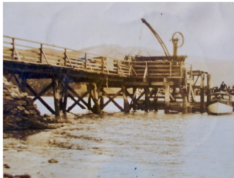
Source: Diamond Harbour & Districts Historical Association Bradley Jetty at Charteris Bay with derrick crane installed by Orton Bradley.
