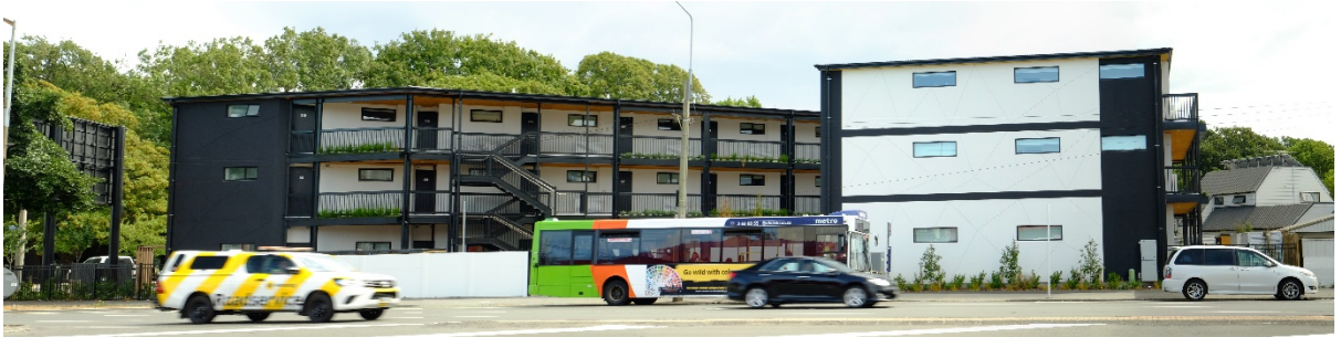
Figure 4: Rear elevation of building labelled A, showing first and second floor access decks and side elevation of building labelled B.
