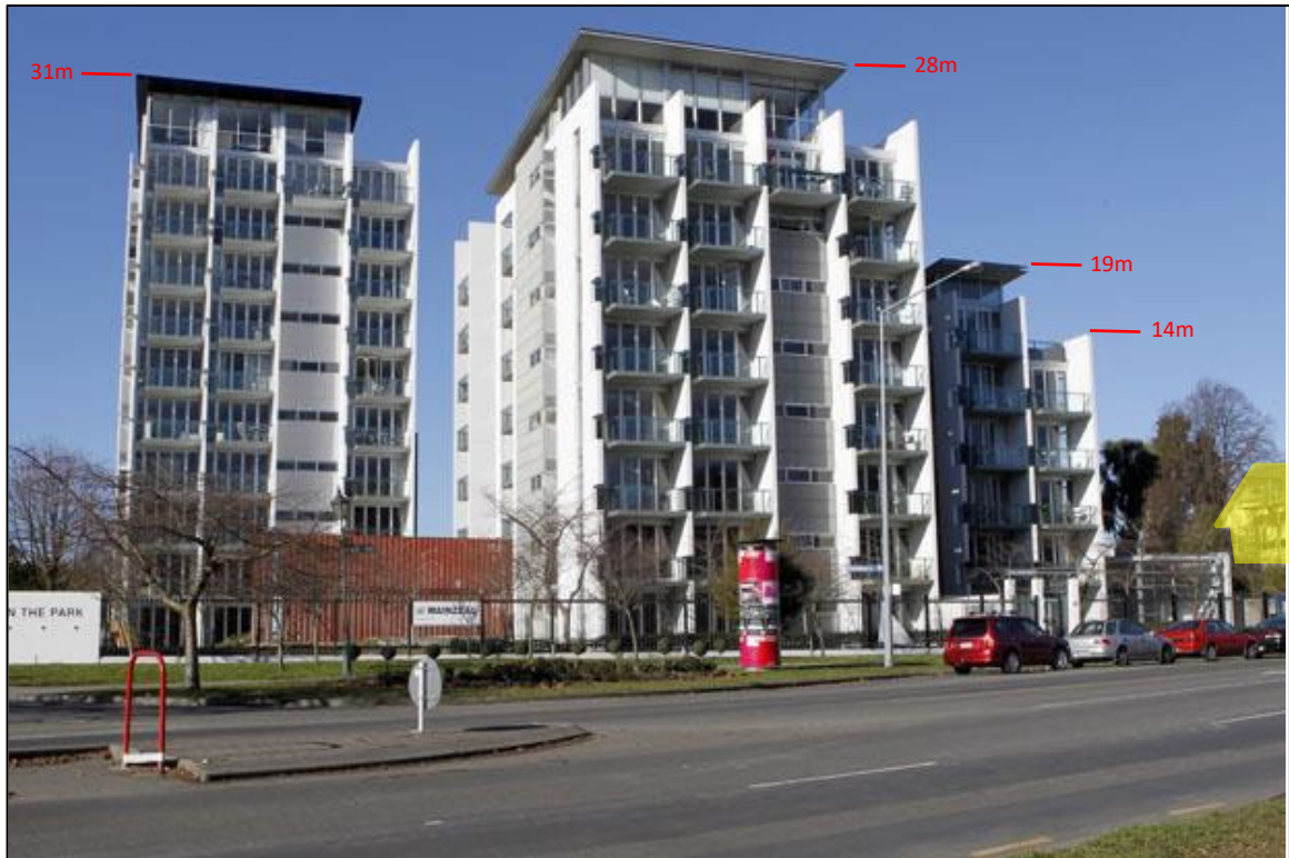
Figure 2: Photo of the Terrace on the Park Apartments as viewed from the west, before their demolition (sourced from Clinton Bird's Statement of Evidence before the Christchurch Replacement District Plan Independent Hearings Panel, dated 14 January 2015). The heights of each building have been indicated in red, along with the location of the Worthington's house in yellow at the right-hand side of the image.
