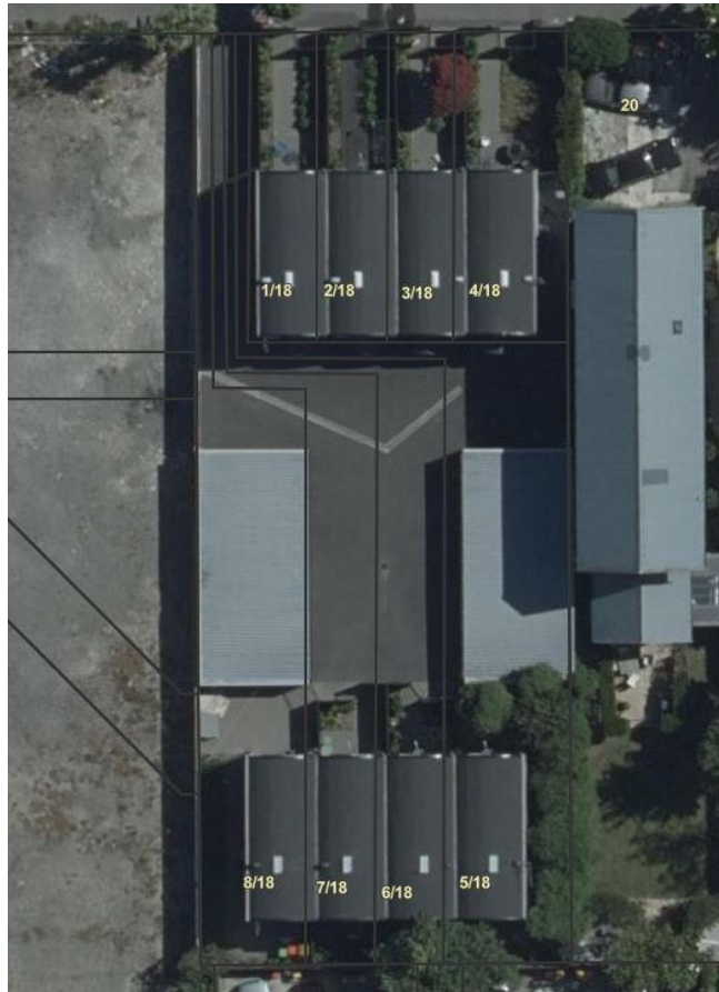
Figure 3: Aerial image of 18 Salisbury Street describing the individual terraced house Unit numbers.
