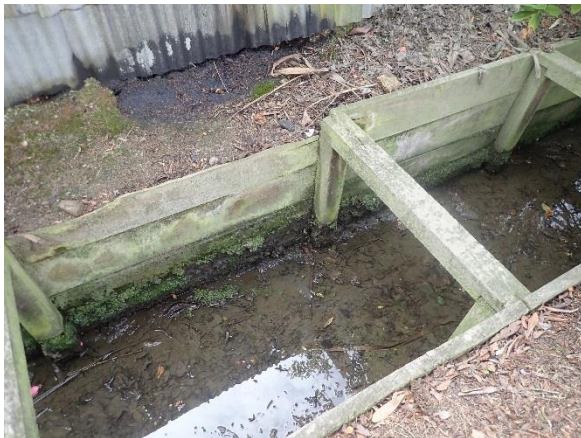
Figure 4. Local ground contamination beside Lydia Street drain. This was sourced to a neighbouring property north of the Foodstuffs site. A hydrocarbon film was also present in the water.
