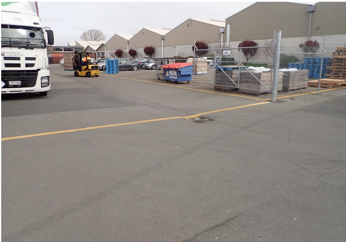
Figure 11. Stormwater drainage from existing busy hardstand areas, which drain to Lydia Street Drain, will be treated to remove contaminants.
