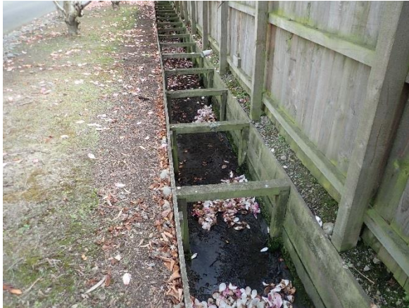
Figure 2. Lydia Street Drain east of Lydia Street. The drain base was wet with a trickling baseflow.
