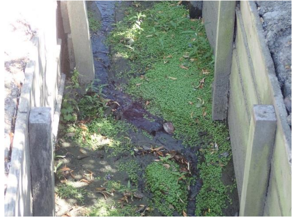
Figure 9. Duckweed and soft sediment in Lydia Street Drain.
