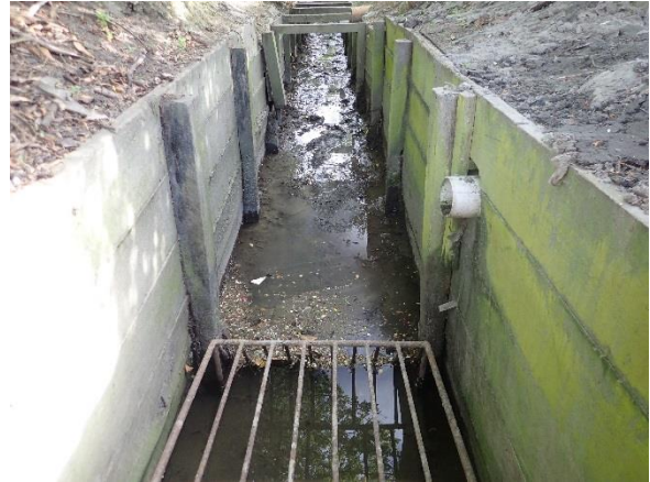
Figure 3. A hydrocarbon film (not from foodstuffs) was evident upstream of the trash rack at Main North Road.
