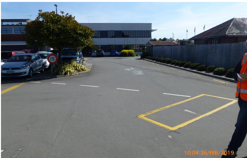
Photograph 4: Lack of pedestrian guidance once in the site.
