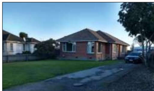
Figure 9. Existing residential building at 161 Main North Road
