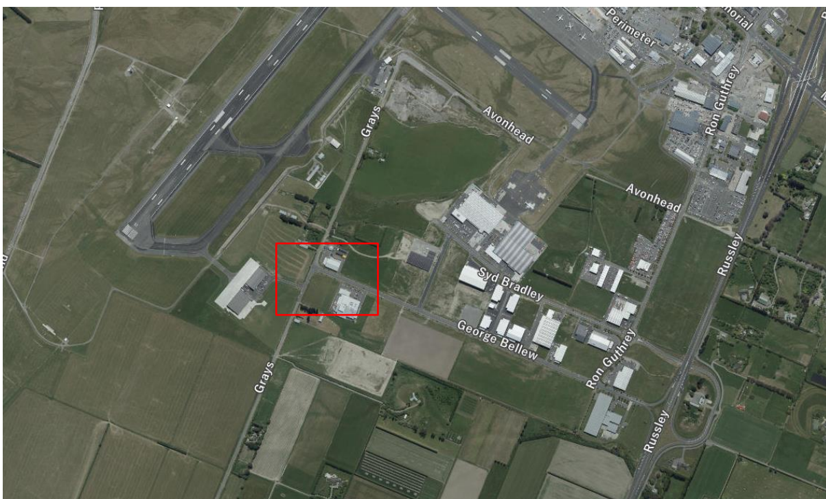
Figure 1: The Intersection of Grays Road and George Bellew Road shown in red.
