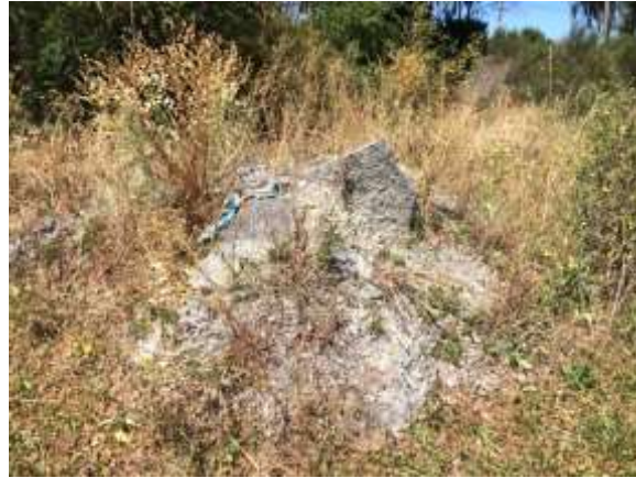
Photo 2: Stockpiled soil with concrete debris
