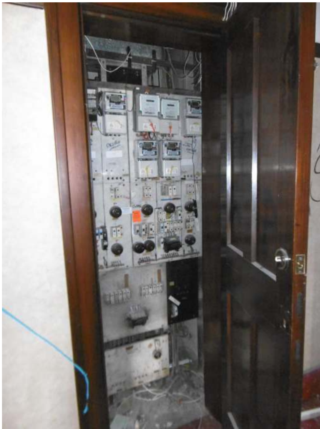
ORIGINAL TYPE SWITCH BOARD CUPBOARD, FIRST FLOOR, WITH MODERN CIRCUIT BREAKERS FITTED
