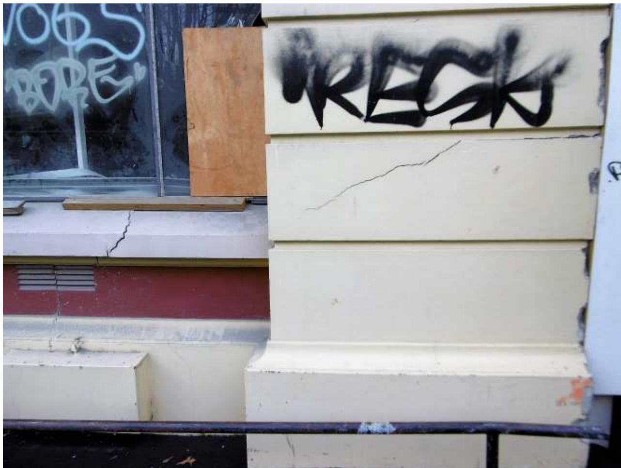
DETAIL OF CRACKING IN THE NORTH EAST CORNER
