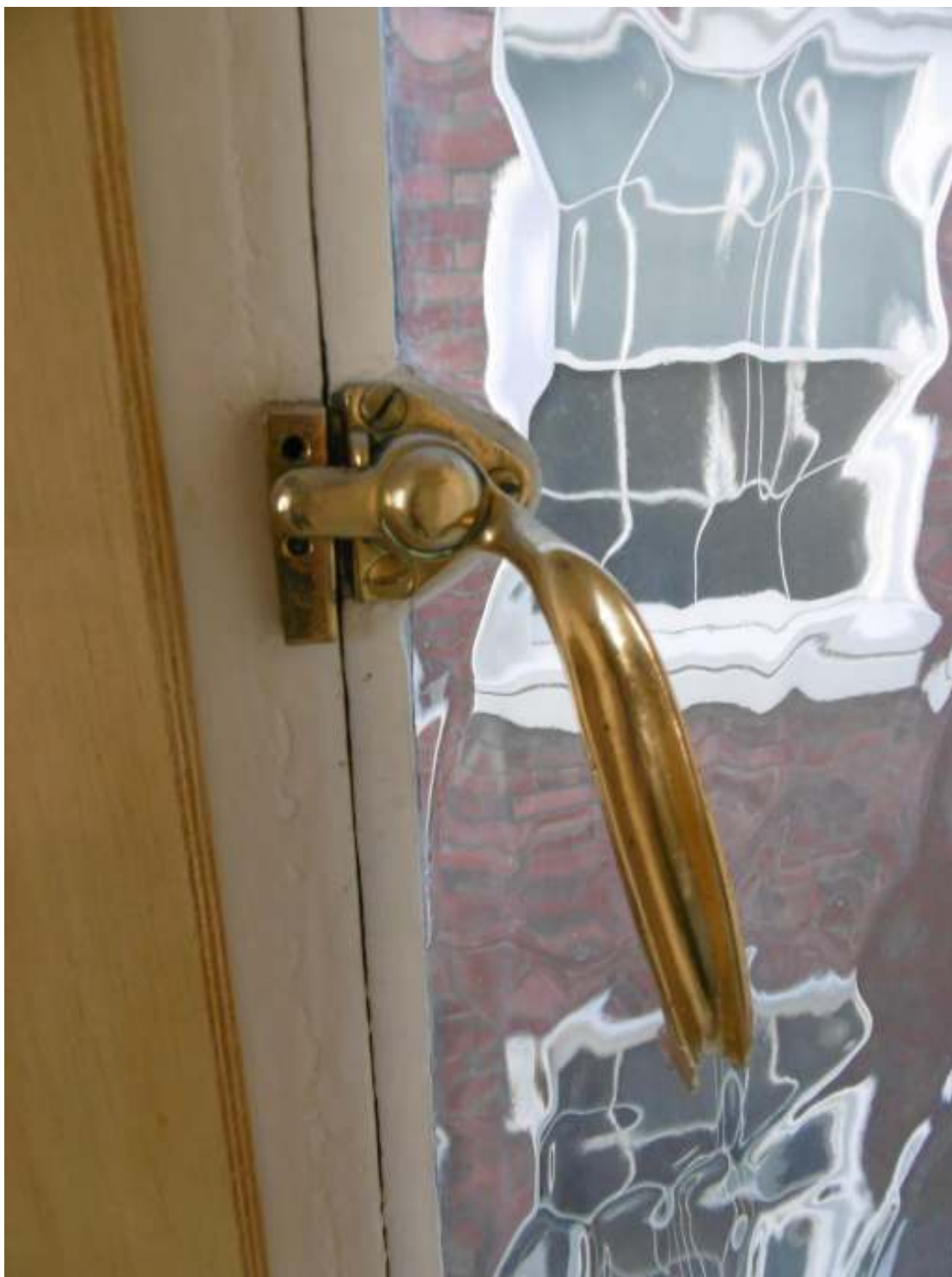
ONE OF THE FEW ORIGINAL BRASS WINDOW CATCHES WHICH REMAIN
