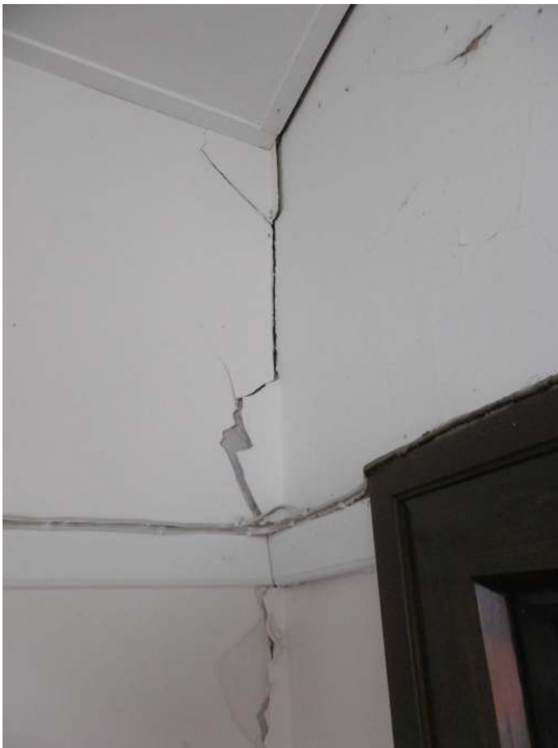
FURTHER WALL SEPARATION BETWEEN THE NORTH AND SOUTH STRUCTURES AT THE GROUND FLOOR
