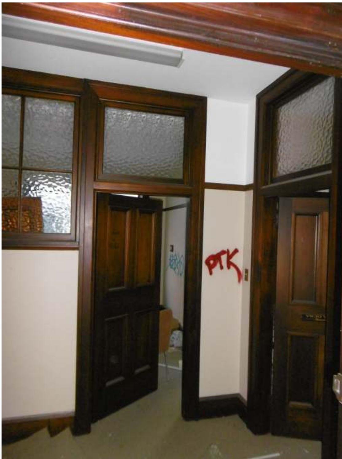
ORIGINAL FIRST FLOOR DOORS, FRAMES AND BORROWED LIGHTS WHICH REMAIN IN GOOD CONDITION
