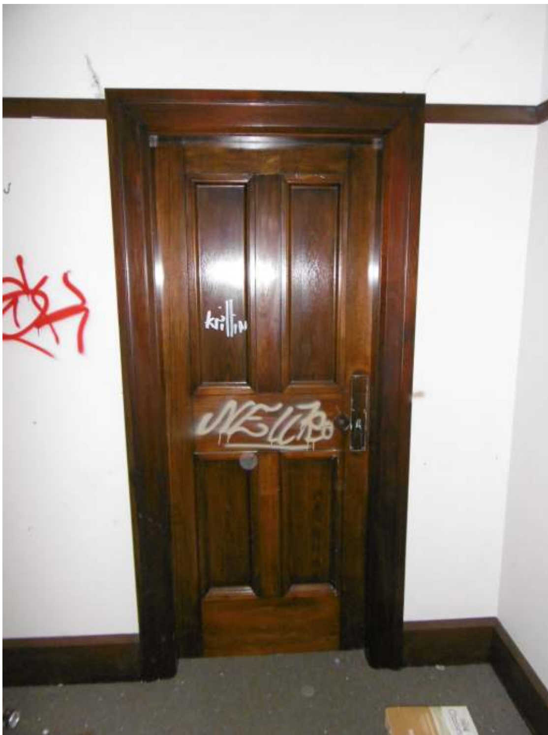
ORIGINAL STAINED TIMBER DOOR AND FRAME, TOP FLOOR
