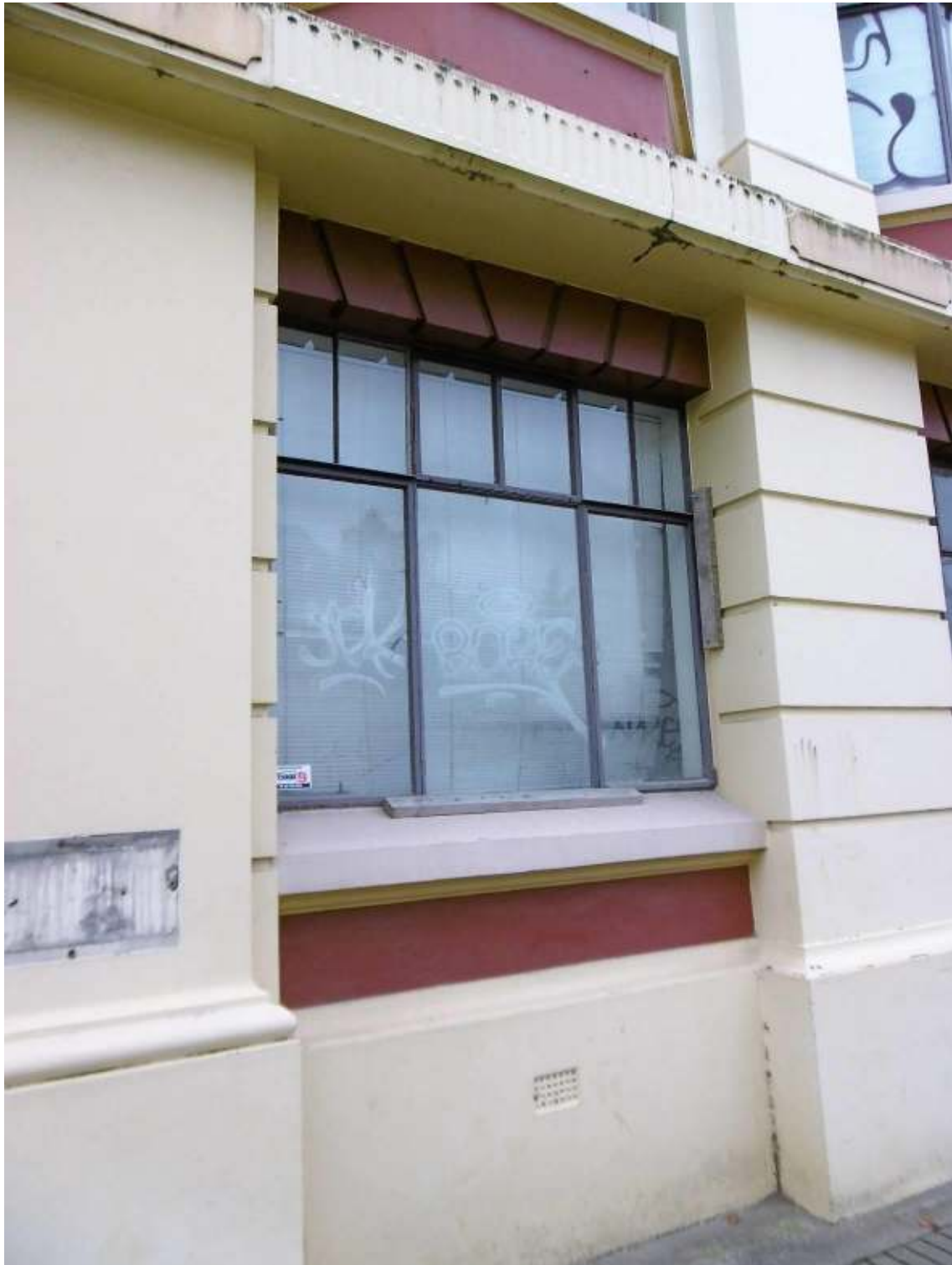
TYPICAL STEEL WINDOW TO THE EAST SIDE OF SOUTH ELEVATION ENTRY DOORS
