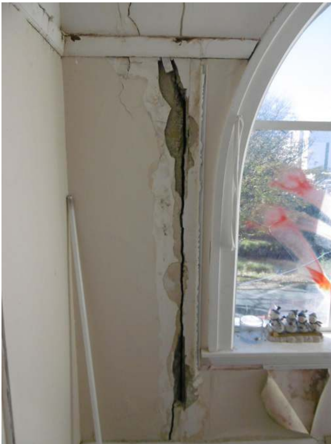
THE VERTICAL GAP IN THE EAST EXTERIOR WALL BETWEEN THE NORTH AND SOUTH STRUCTURES, AT THE FIRST FLOOR, CAUSED BY THE EARTHQUAKE EVENT
