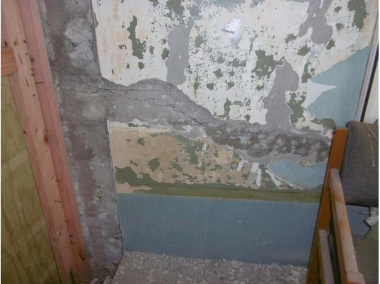
DETAIL OF NORTH EAST CORNER COLUMN CRACKING
