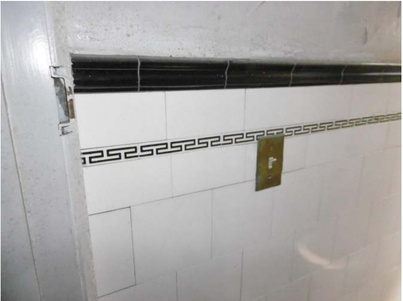
EXTANT TOILET AREA TILING, TOGETHER WITH ORIGINAL BRASS LIGHT SWITCH PLATE.
