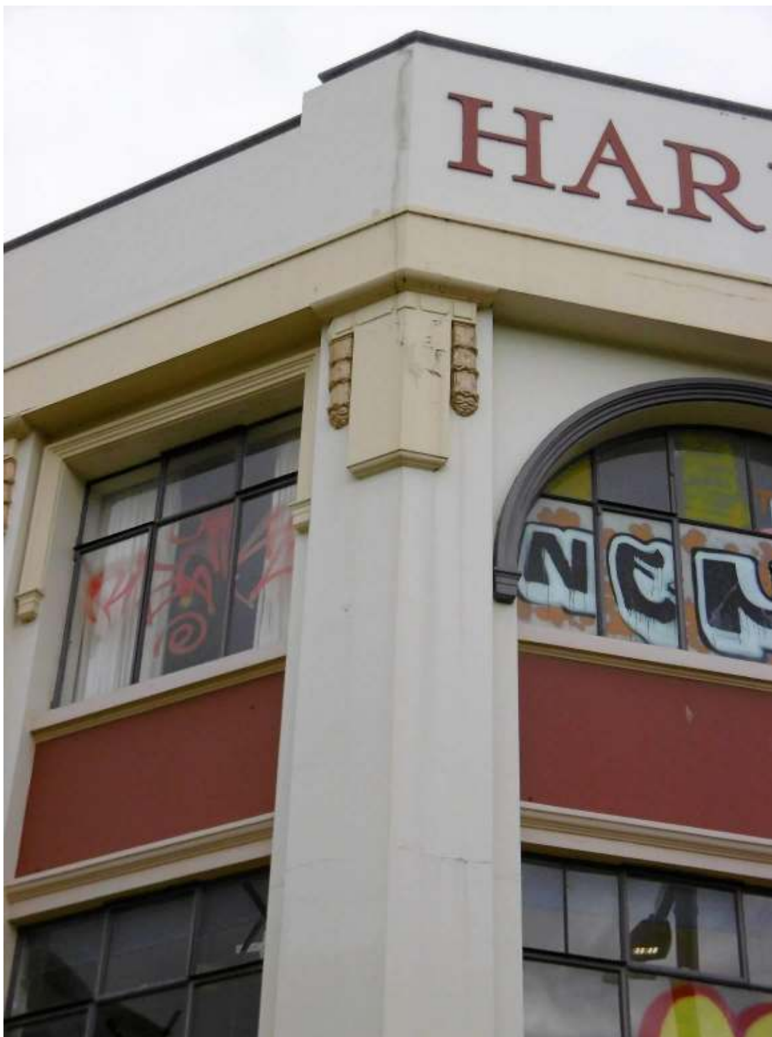
UPPER DETAIL OF THE SOUTH EAST CORNER, SHOWING CRACKING TO THE PARAPET
