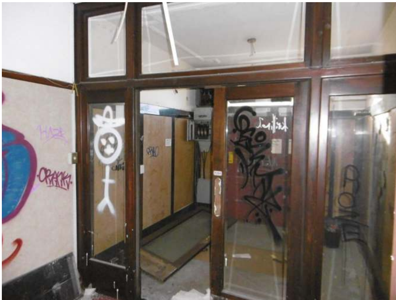
TIMBER DOOR SET AND FRAME, FROM THE MAIN STAIR, LOOKING TOWARDS THE ENTRANCE FOYER
