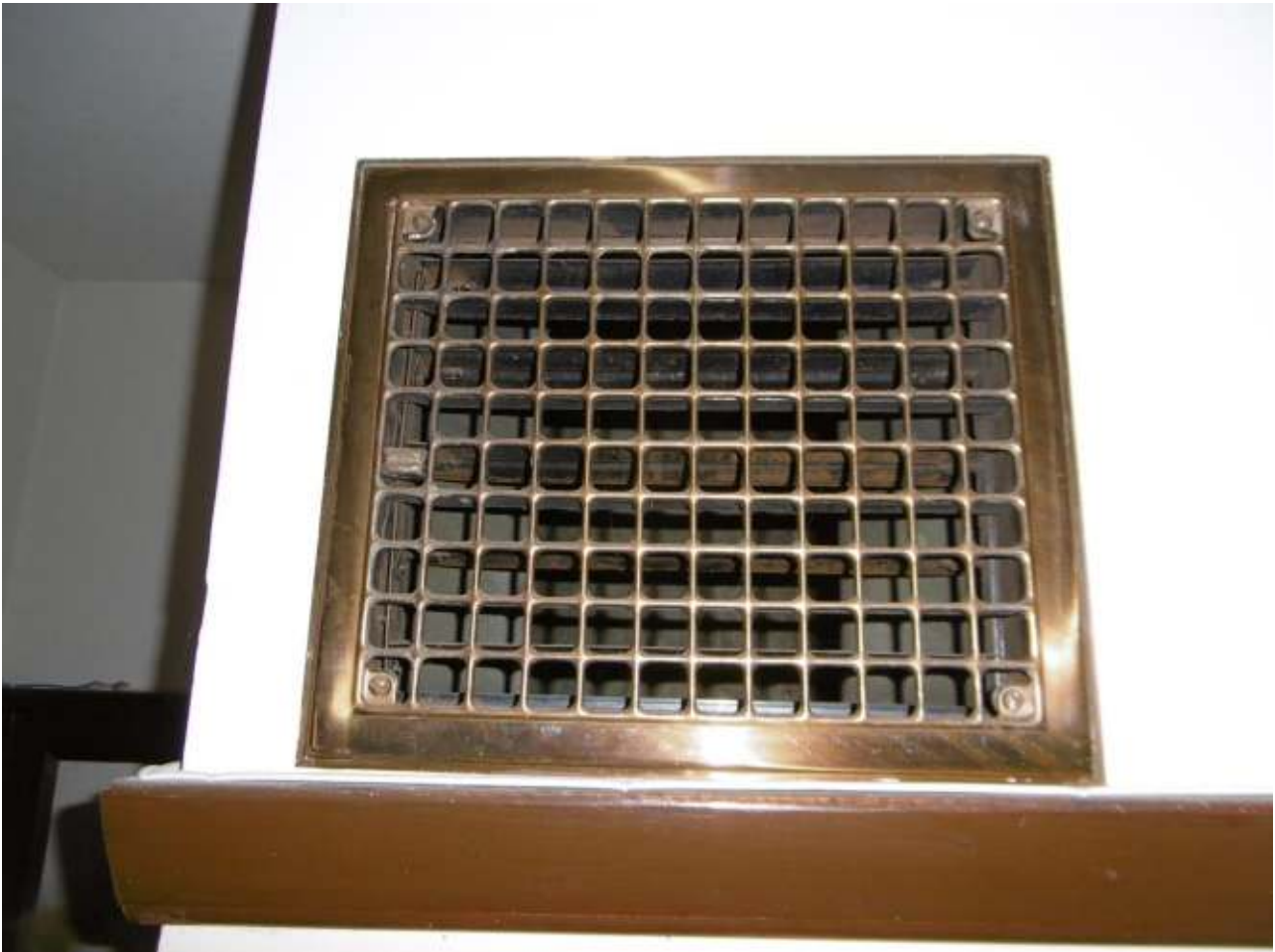
ORIGINAL BRONZE WALL GRILL, WHICH WAS PART OF THE TEMPERED AIR VENTILATION SYSTEM.
