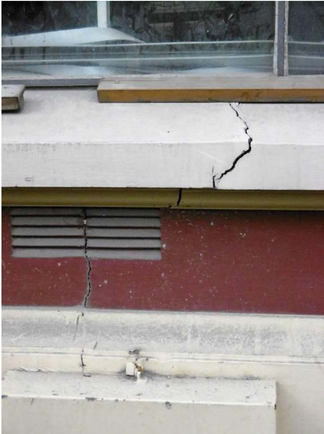
CLOSE-UP OF EARTHQUAKE INDUCED CRACKING TO THE SILL AND INFIL PANEL BELOW THE WINDOW, NORTH EAST CORNER OF HARLEY BUILDING
