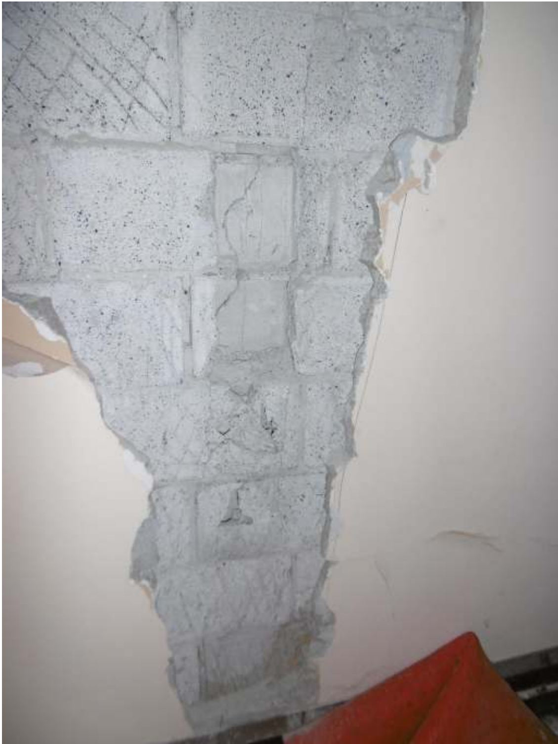
TYPICAL INNES BELL BLOCK INTERIOR WALL, GROUND FLOOR, SHOWING EARTHQUAKE INDUCED CRACKING
