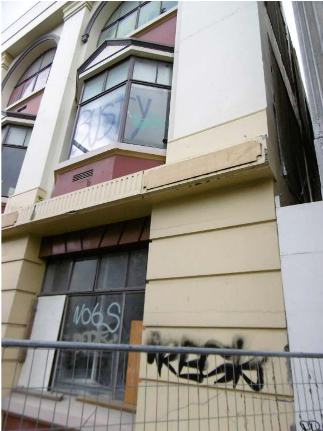
GENERAL VIEW OF NORTH EAST CORNER COLUMN, SHOWING HORIZONTAL CRACKING IN THE PLASTER WORK, AND CORRUGATED IRON COVERING THE DEMOLISHED PANELS IN THE NORTH WALL
