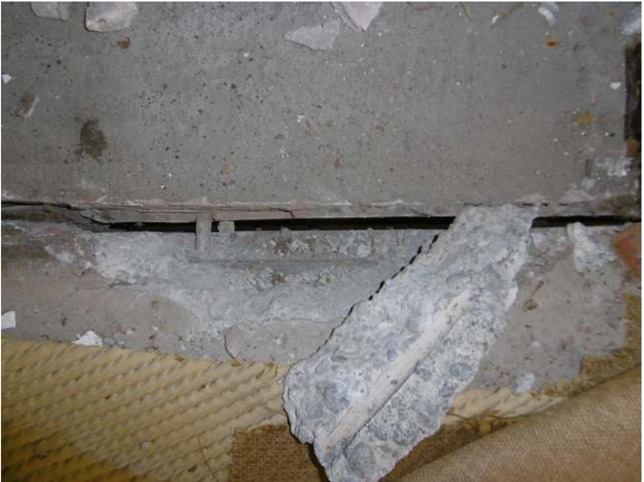
THE GAP IN THE FLOOR BETWEEN THE NORTH AND SOUTH STRUCTURES, AT THE FIRST FLOOR, CAUSED BY THE EARTHQUAKE EVENT
