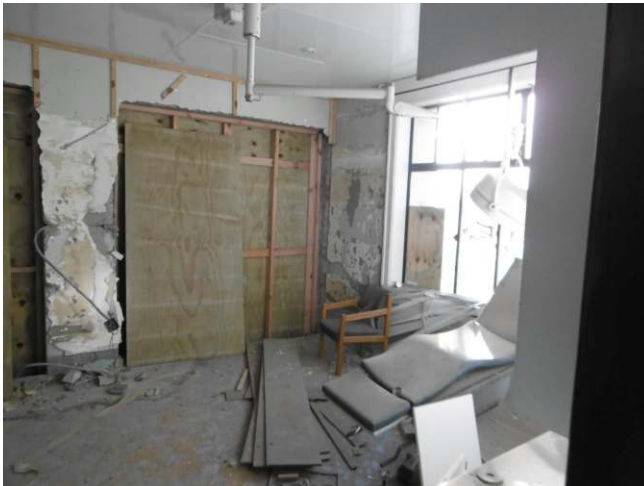
INTERIOR OF NORTH EAST CORNER OF BUILDING, GROUND FLOOR, SHOWING COLUMN CRACKING AND BRICK INFILL PANELS REMOVED
