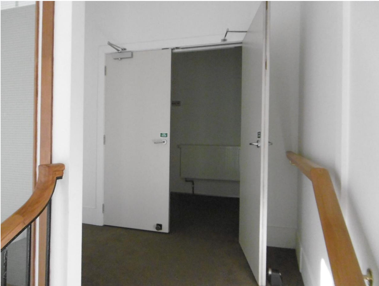
UPPER FLOOR STAIR FOYER FROM THE STAIRS. NOTE THE MODERN SMOKE STOP DOORS. THE ORIGINAL TIMBER HANDRAIL IS ON THE LEFT, WITH A MODERN ONE ON THE RIGHT.
