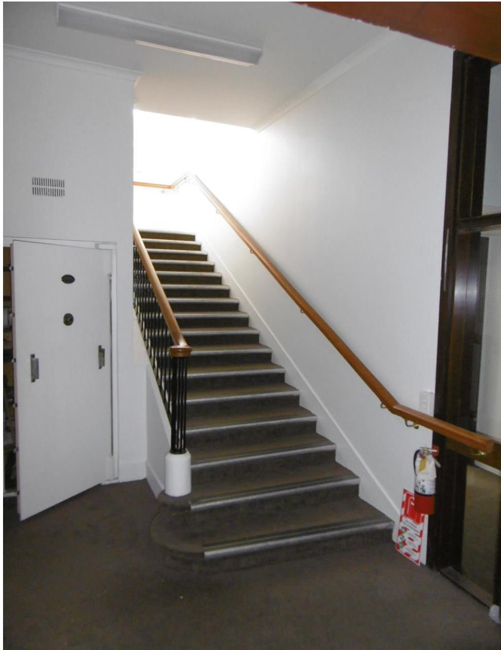
CENTRAL STAIRWAY WITH ORIGINAL STEEL BALUSTRADE AND TIMBER HANDRAIL ON THE LEFT HAND SIDE.
