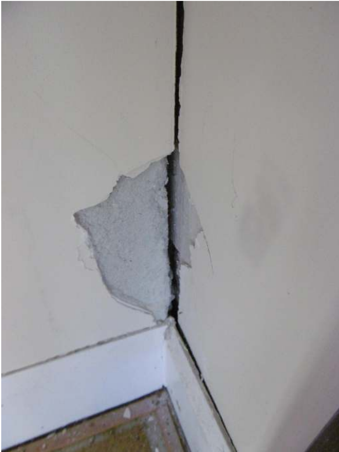
WALL SEPARATION BETWEEN THE NORTH AND SOUTH STRUCTURES AT THE GROUND FLOOR
