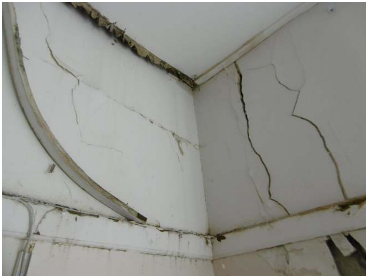
UPPER WALL DAMAGE COUSED DURING THE EARTHQUAKE EVENT
