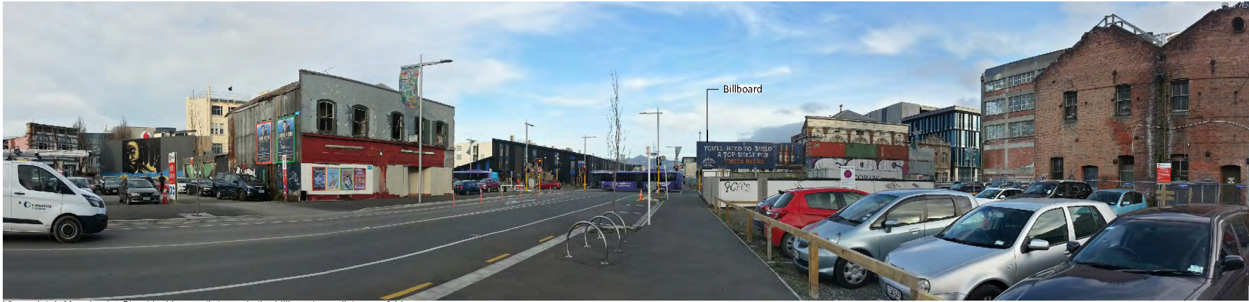
Viewpoint 4, Manchester Street looking south towards the billboard at a distance of 44 m
