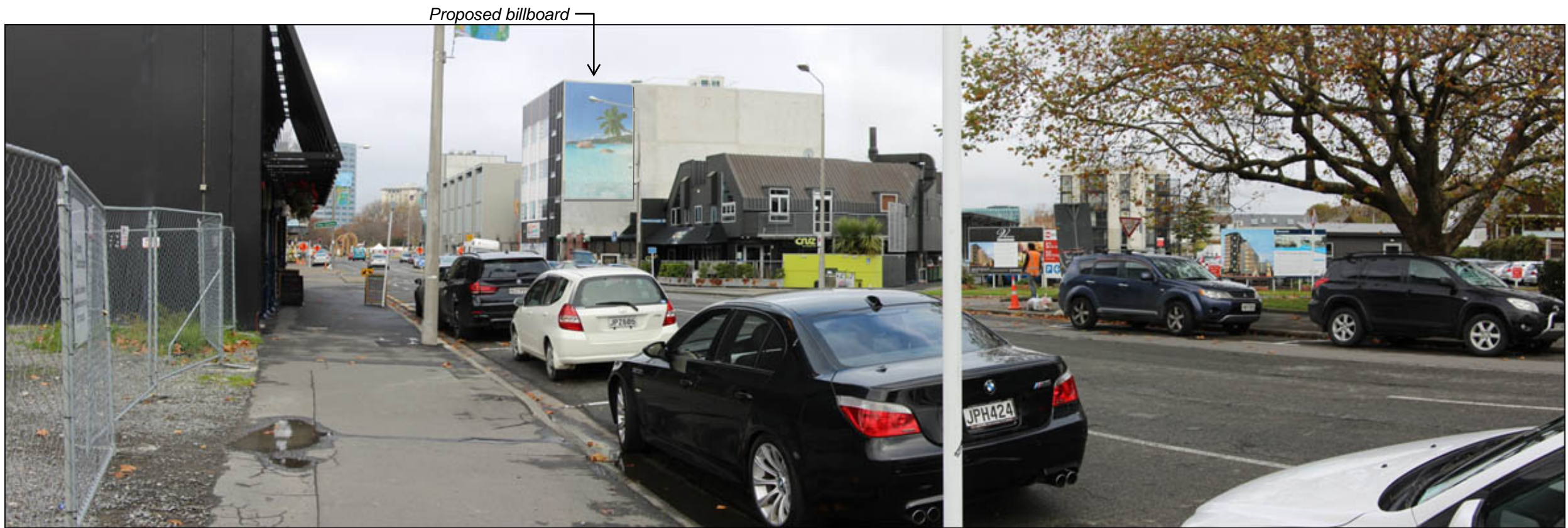
Photograph 1 From the west side of Victoria Street the proposed sign is fully apparent. Note that it occupies a relatively small portion of the façade to which it is attached.
