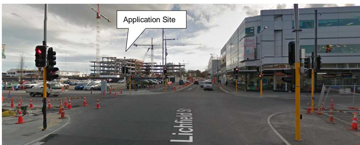
Figure 8: Street View of Intersection, Lichfield Street Westbound
