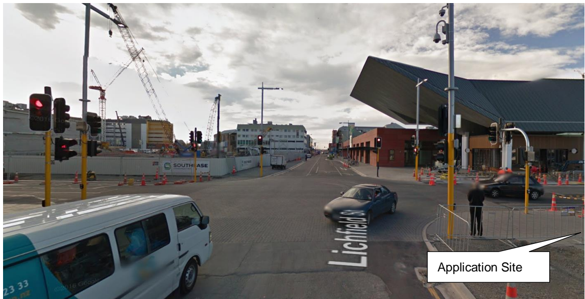
Figure 9: Street View of Intersection, Lichfield Street looking east
