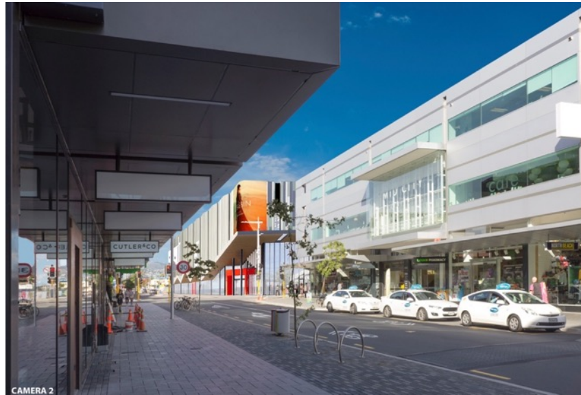
Figure 79: A view of the screen on the top left hand and top right hand corners of the northern and eastern elevations of the EntX Building respectively, as seen from the opposite side of the road just south of the first floor level pedestrian bridge over Colombo Street.
