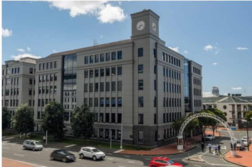
Figure 49: Maritime Square, Viaduct Harbour, Auckland.
