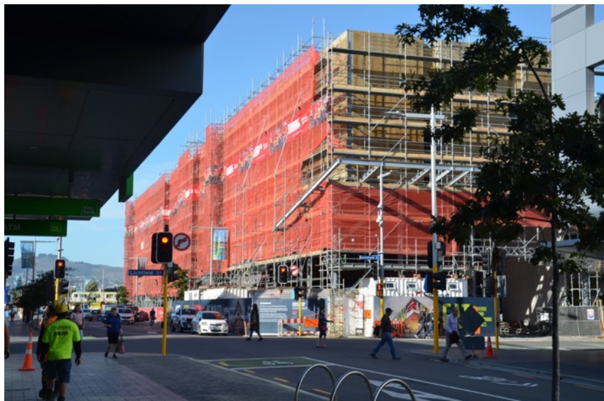
Figure 14: A view of the inclined steel frame for the veranda (under construction), illustrating how from various viewpoints it will obscure the lower portions of the proposed corner-mounted EntX digital screen above it.
