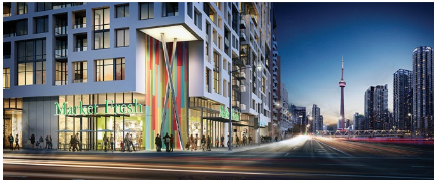
Figure 53: A 'recessed' corner building in the USA.
