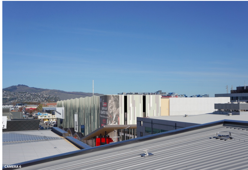
Figure 83: A view of the screen wrapping around the north-eastern corner of the EntX Building, as seen from the rooftop terrace of the proposed but yet to be fitted out single apartment on the roof of The Crossing building.
