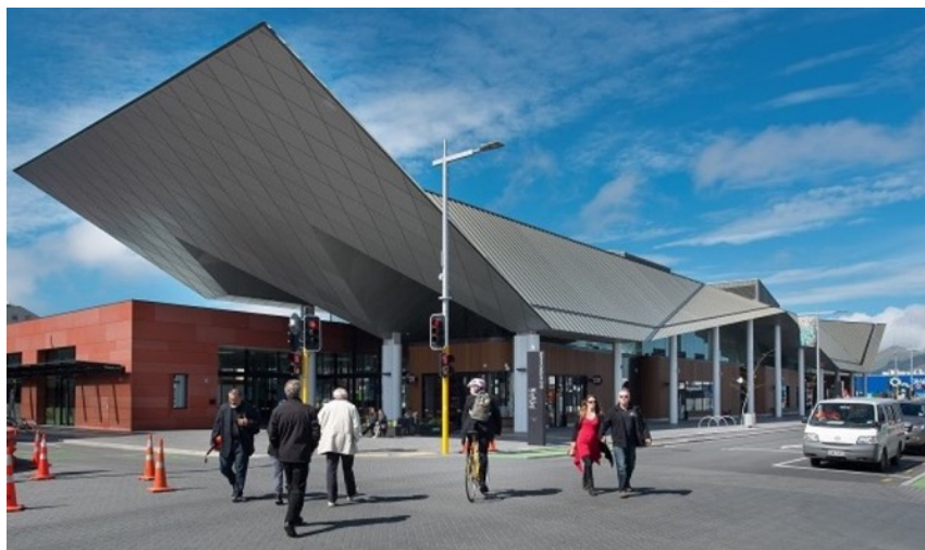
Figure 28: A view of the main entry/exit of the bus interchange on Colombo Street (right) and Lichfield Street (left).
