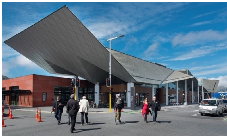
Figure 5: The large Christchurch Bus Interchange Building , viewed from the north-west corner of Colombo (to the right of the image) and Lichfield Street (to the left of the image), looking south-east towards the main Interchange entry.
