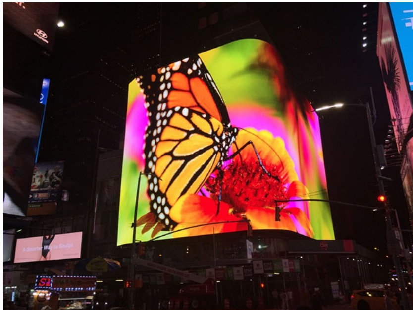
Figure 66: A digital screen forming an inextricable component of the form of a building (location unknown).
