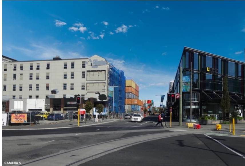
Figure 82: A very distant view of the screen wrapping around the corner of the EntX Building, as seen from the opposite side of the road near the intersection of Lichfield Street East and High Street.
