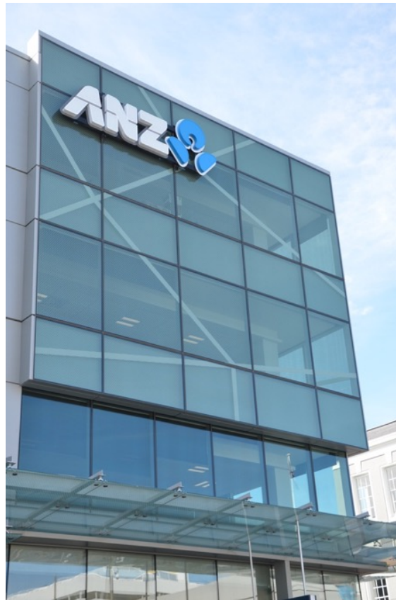
Figure 8: The new four storey ANZ Bank building on the eastern side of Colombo Street, just to the north of Cashel Street
