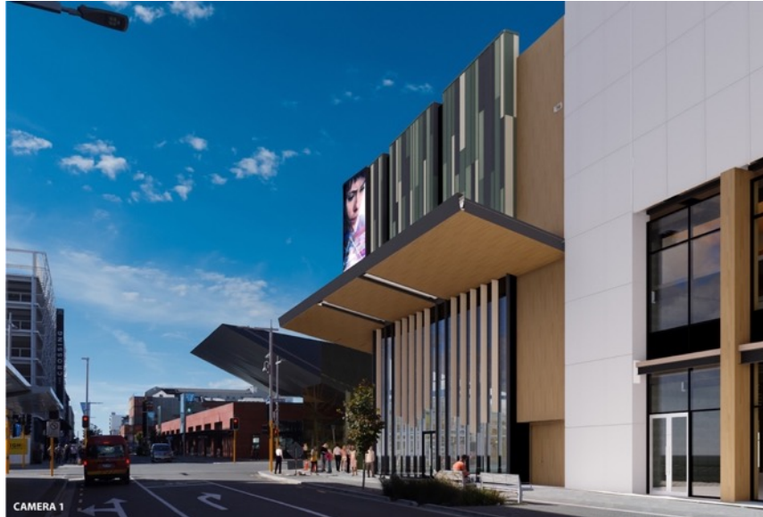
Figure 78: A view of the screen on the top left hand corner of the northern elevation of the EntX Building, as seen from the opposite side of the road near the western end of Lichfield Street.
