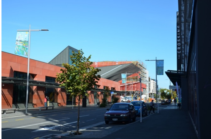
Figure 26: A view looking west along the northern side of Lichfield Street towards Colombo Street, illustrating the juxtaposition of the Bus Interchange's large scale sloping entrance canopy, read against the background of the EntX building.
