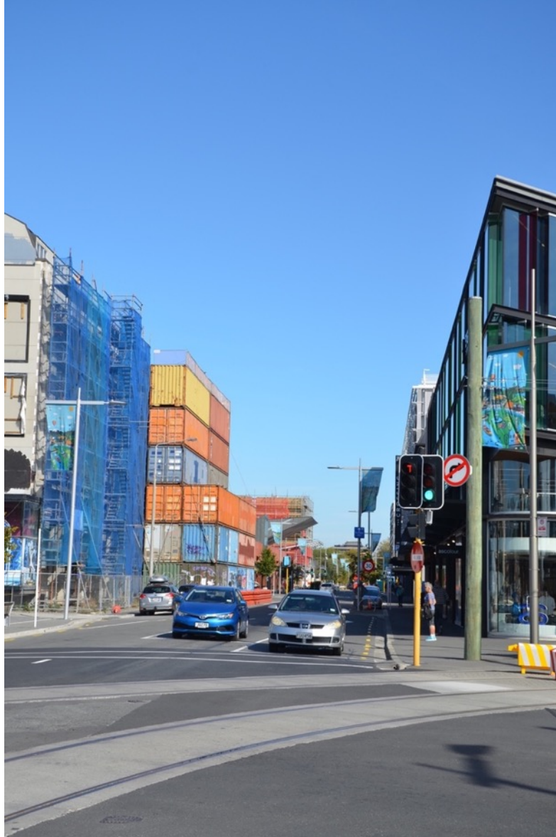
Figure 22: The view of the EntX building corner from the footpath on the north-western corner of the East Frame. The sign on the corner will be barely visible because it will be largely obscured by the cantilevered canopy over the entry to the Bus Interchange. It should also be noted that currently the Lichfield Street frontage is not activated because of the state of the buildings on its southern side. Once these buildings are redeveloped or refurbished, there will be more visual interest to reduce any visual impact the screen may initially have.
