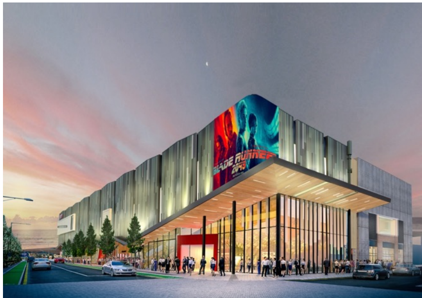
Figure 68: The proposed digital screen acting as cladding to the corner element of the EntX building. The screen is not unlike a smaller version of the cube form illustrated in Figure 67 above.
