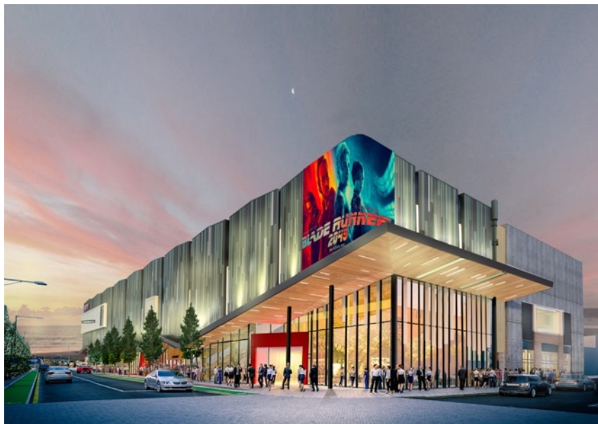
Figure 56: The EntX Building, currently under construction in Christchurch.
