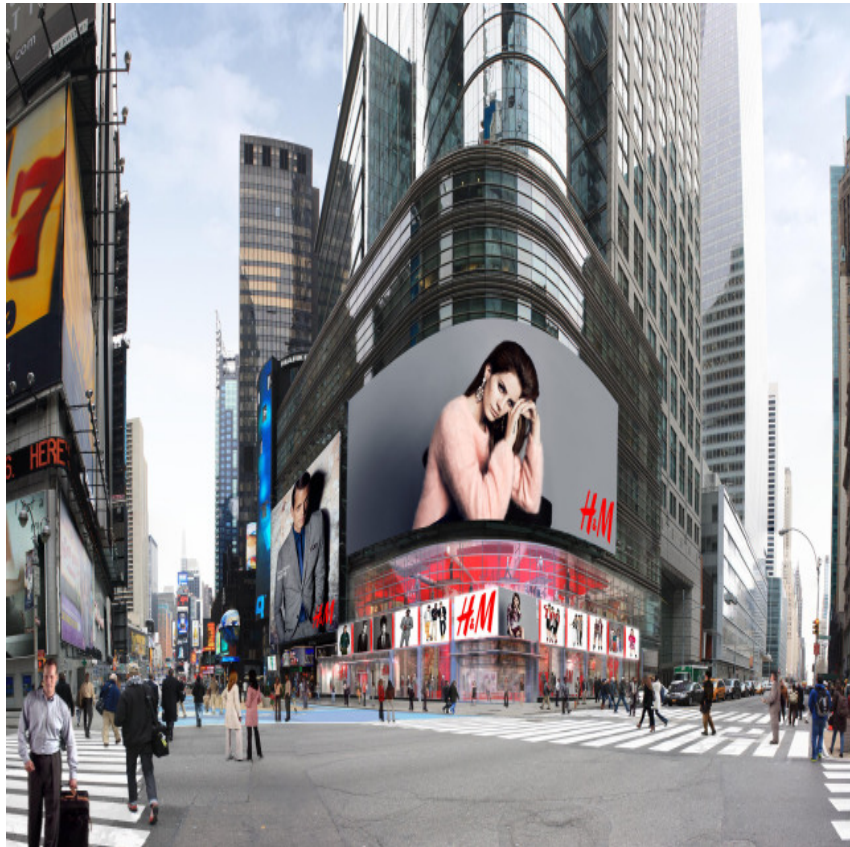
Figure 65: A large screen wrapped around the upper levels of the curved corner component of a building in New York.
