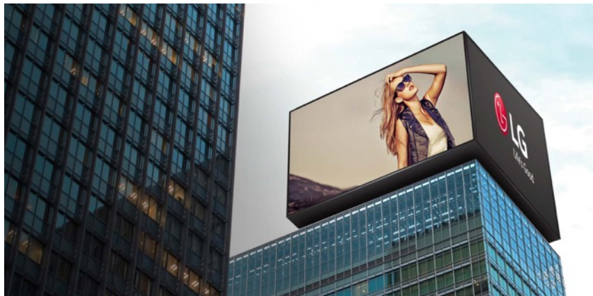
Figure 64: A digital screen, in the USA, wrapped around a 'floating' rectangular form which is expressed as a distinct component within the overall composition of the building.
