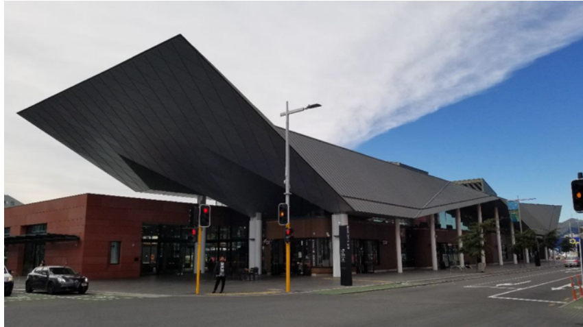
Figure 39: The Bus Interchange building, viewed for the north -west corner of Colombo and Lichfield Streets (source: John Lonink’s evidence).
