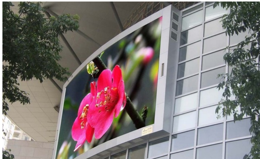
Figure 60: A screen on an office building in Berlin.
