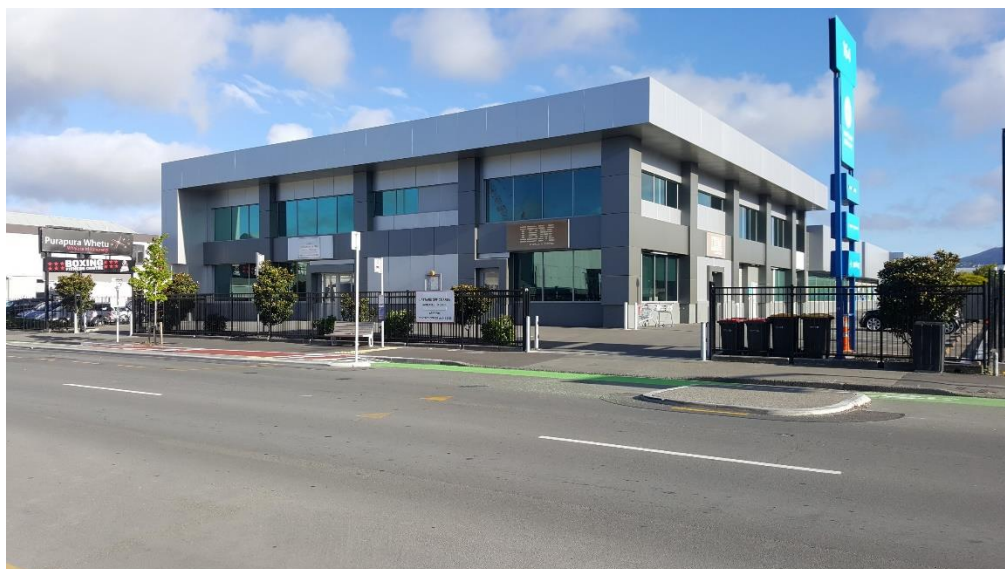
Photograph 7: Wide Driveway Gap at Cyclist Accident Site
