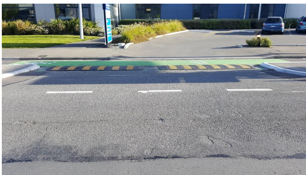
Photograph 6: Speed Humps at Police Station Driveway
