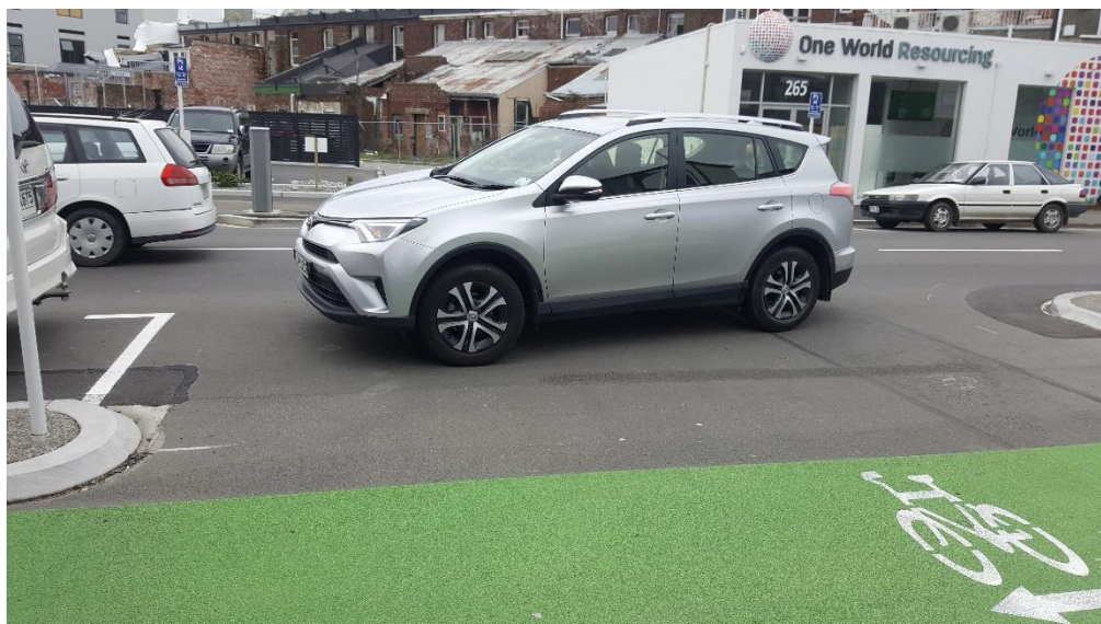
Photograph 2: Car Drop-off Intrudes into Traffic Lane (even without downstream build-out)
