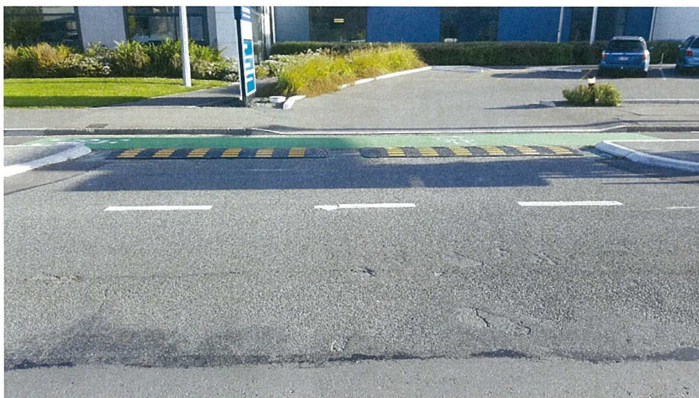
Photograph 6: Speed Humps at Police Station Driveway
