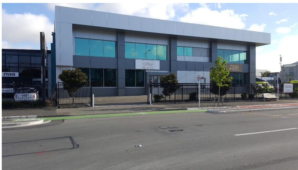
Photograph 4: Upstream Build-out Set Back
