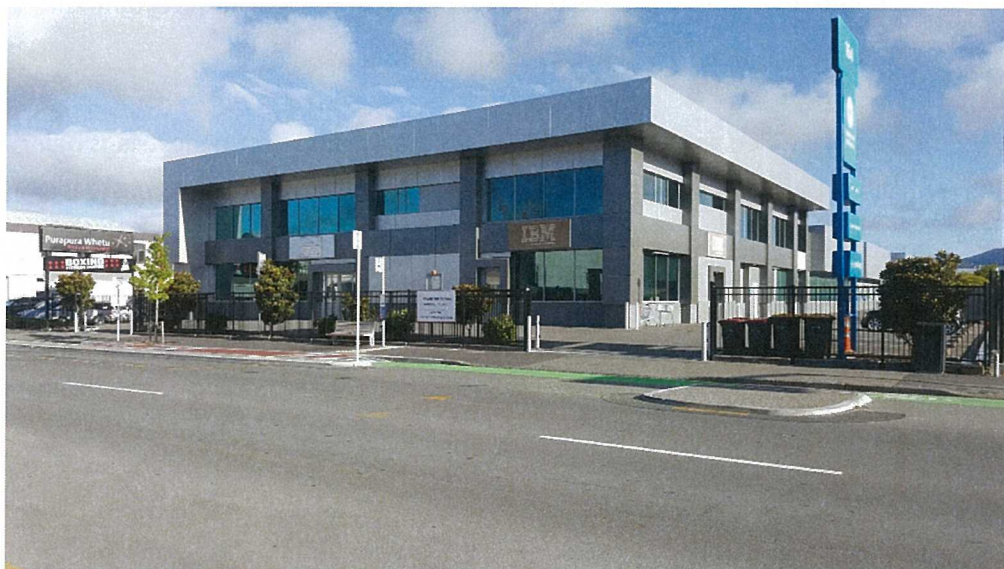
Photograph 7: Wide Driveway Gap at Cyclist Accident Site
