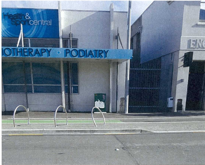
Photograph 1: Damaged Cycle Stand
