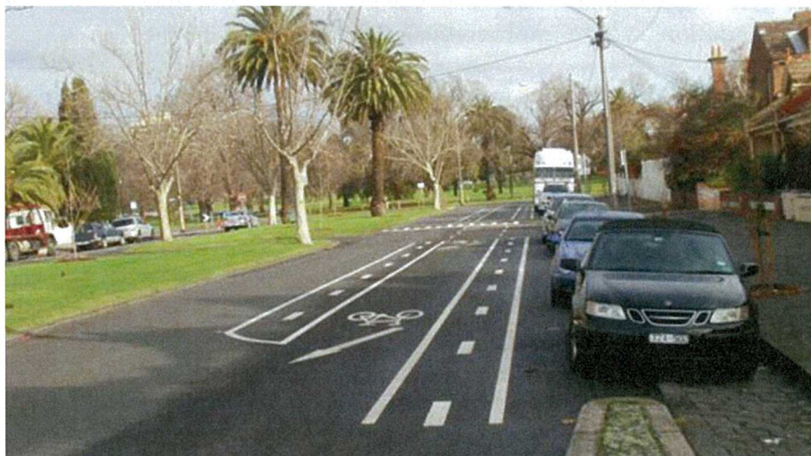
Figure 4.5: A bicycle/car parking lane with painted separators between cyclists, parked cars and the traffic lane
