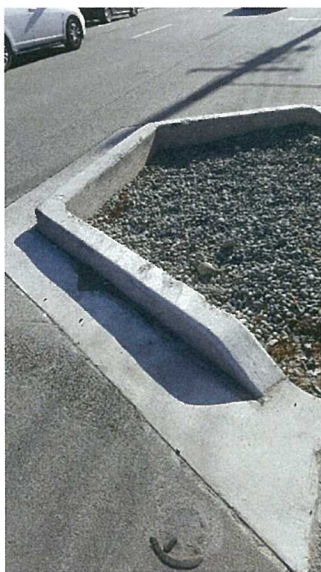
Photograph 5: Tree Pit Collision Evidence
