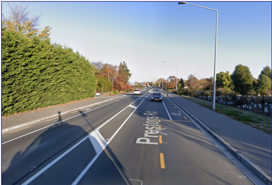
Figure 6: View looking west of the existing Prestons Road carriageway layout from outside the proposed western car park access. (Source = Google Streetview).
