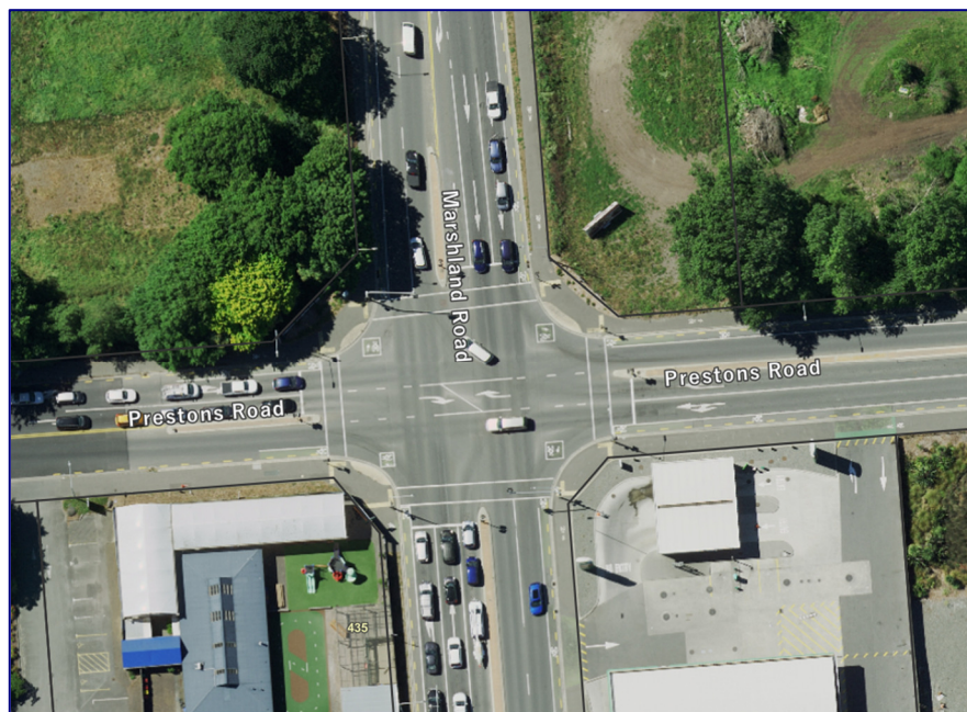
Figure 10: Existing layout of the signalised Marshland/Prestons intersection located 330m west of the application site
