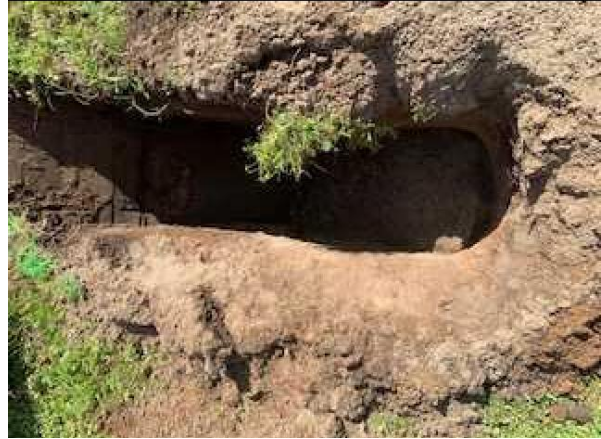
31.0 Test Pit – Prestons Road
