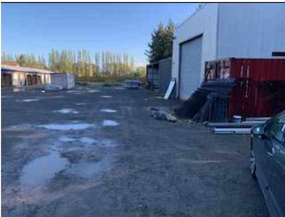
17.0 394 Prestons – Building east boundary
