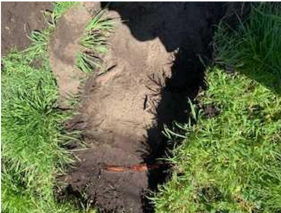
27.0 Test Pit – Prestons Road
