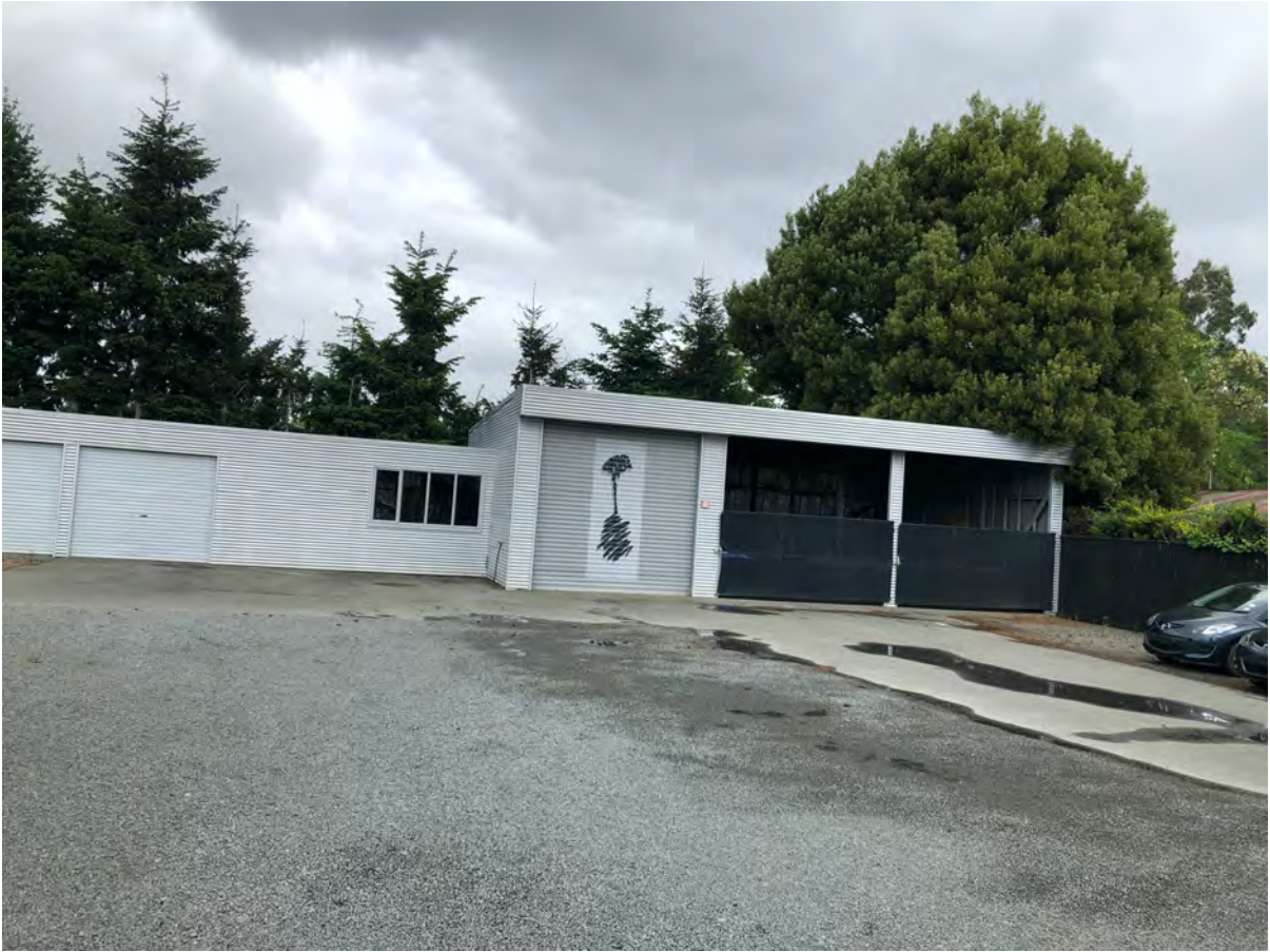
Figure D-1. Large utility building at 404-406 Prestons Road.
