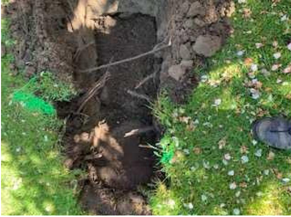
30.0 Test Pit – Prestons Road
