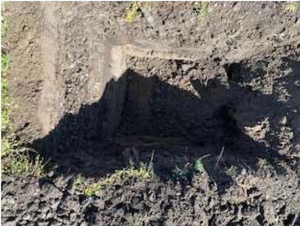
23.0 Test Pit – Prestons Road
