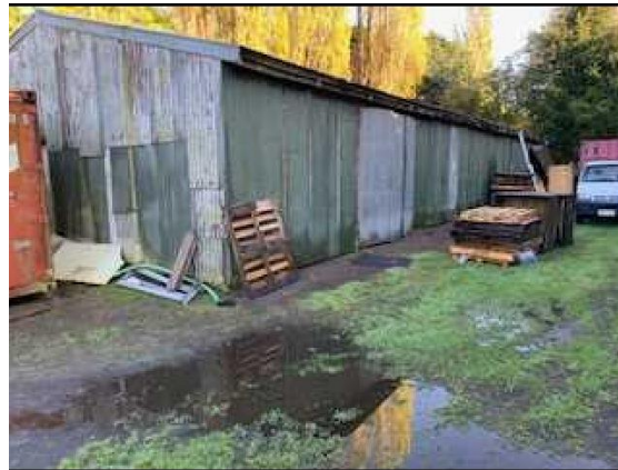
2.0 390 Prestons – Rear workshop (Storage Building)
