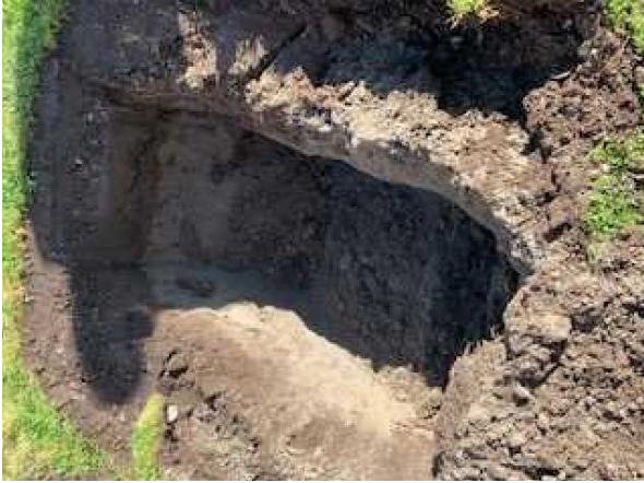
19.0 Test Pit – Prestons Road
