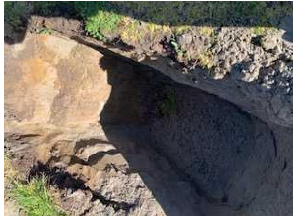
22.0 Test Pit – Prestons Road
