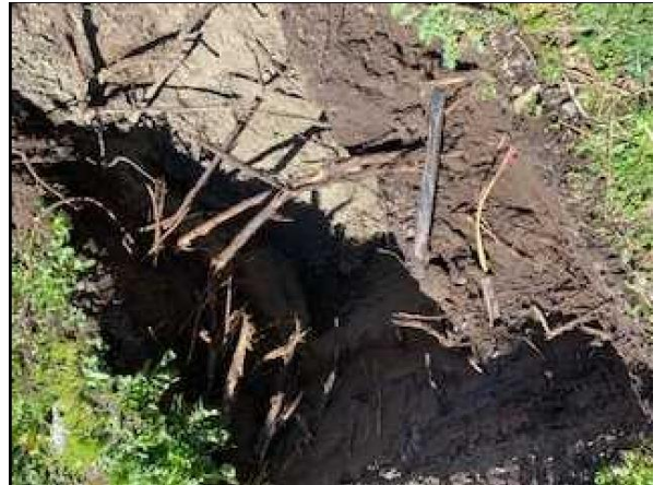
24.0 Test Pit – Prestons Road
