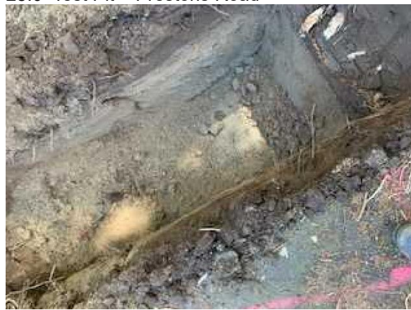
30.0 Test Pit – Prestons Road
