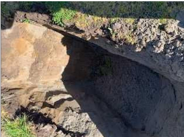
21.0 Test Pit – Prestons Road
