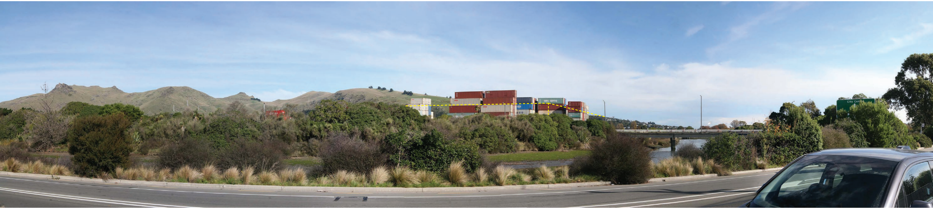
Photographic viewpoint 1 from outside 869 Ferry Road looking southwest to site. Note containers stacked as high as approximately 15.6 m (6 containers). Note maximum building height of 11 m from the paved surface / 4.2 containers (dotted yellow line). At the permitted height, more of Montgomery Spur is visible. The Proposal will also extend the built form further right into the greenspace area. Photograph by J.Head 8 May 2023 (50 mm focal length with images stitched to form panorama).
