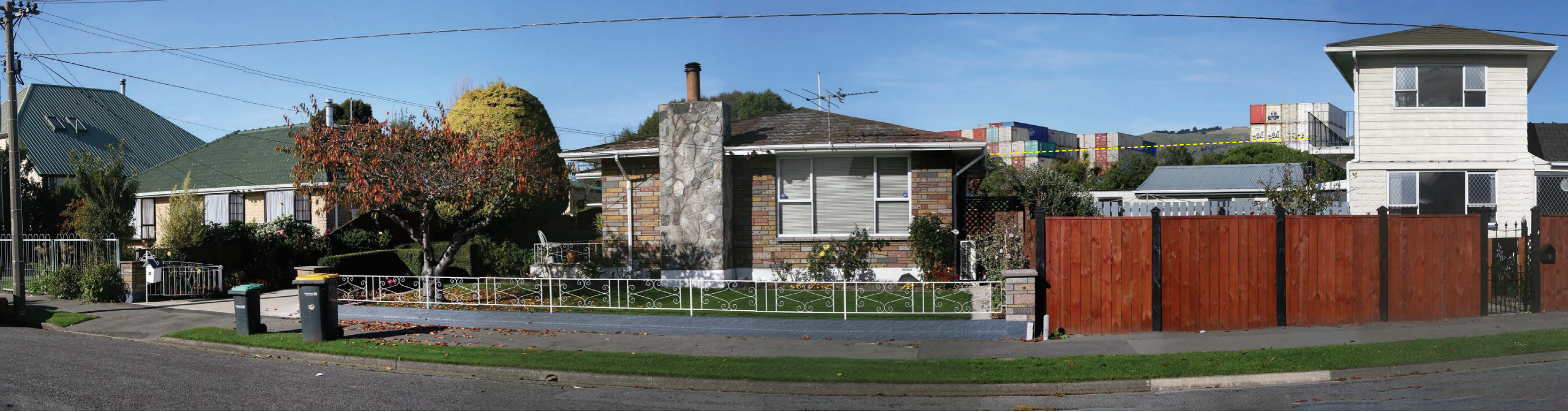
Photographic viewpoint 5 from outside 35 Gould Crescent looking southwest to site. Note maximum height of 11 m from the paved surface / 4.2 containers (dotted yellow line). Photograph by J.Head 8 May 2023 (50 mm focal length with images stitched to form panorama).
