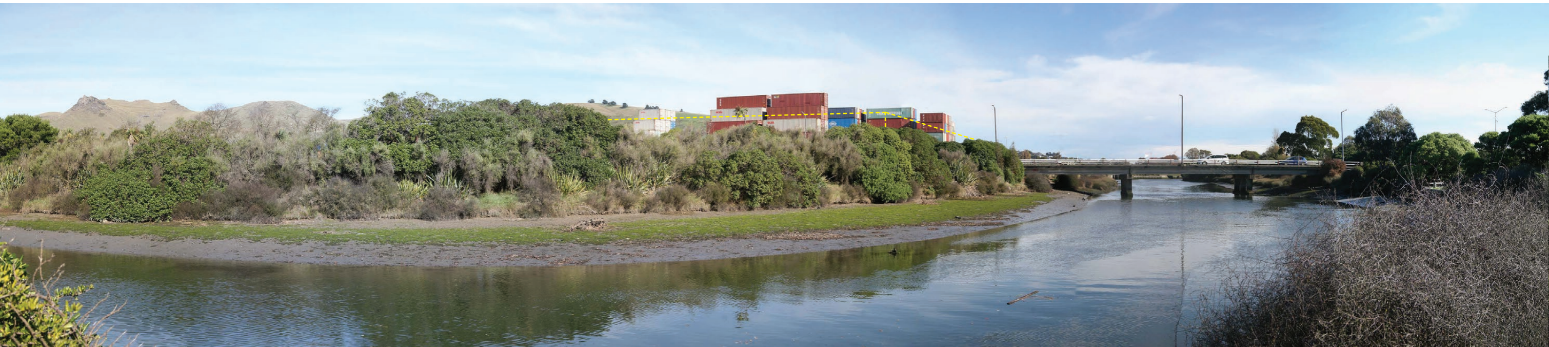
Photographic viewpoint 2 from Tow Path public track looking southwest to site. Note maximum building height of 11 m from the paved surface / 4.2 containers (dotted yellow line), where the existing native planting provides an effective buffer to these views. The Proposal also extends the built form further right into the greenspace area. Photograph by J.Head 8 May 2023 (50 mm focal length with images stitched to form panorama).
