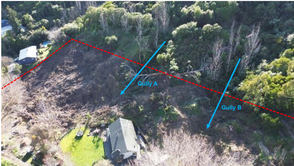
Figure 4: Aerial view of the site looking northeast. Major gullies approximately marked in blue
