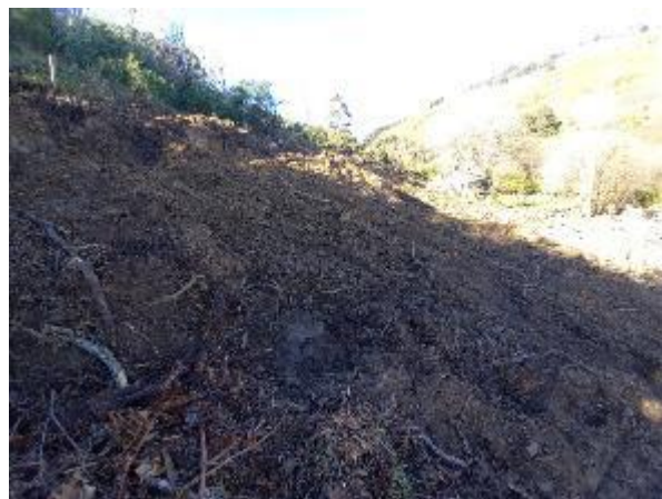
Figure 10: View along the east boundary of the site from near the north end, looking south
