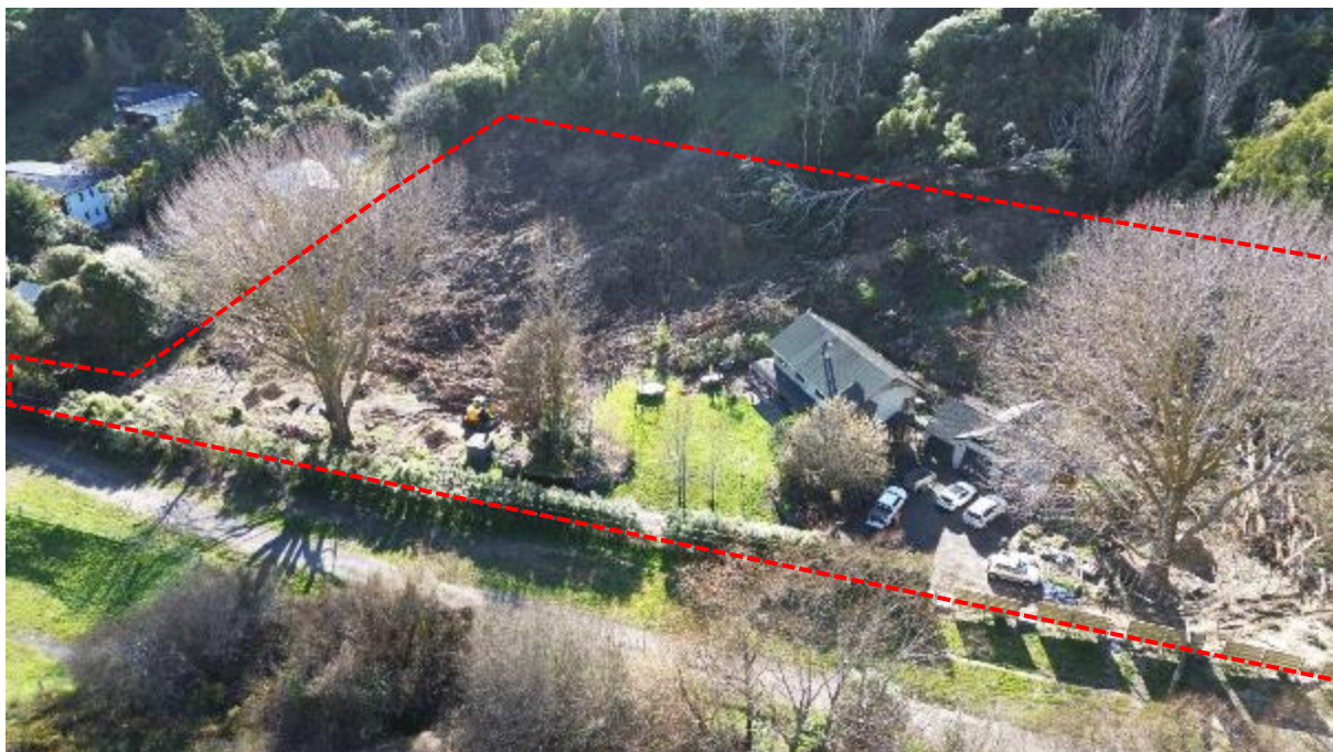
Figure 5: Aerial view of the site looking east
