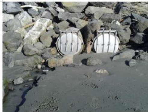
Figure 2. Burgess Street outfall in May 2014
