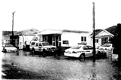
The Sumner Police Station became the Sumner Civil Defence H.Q.
