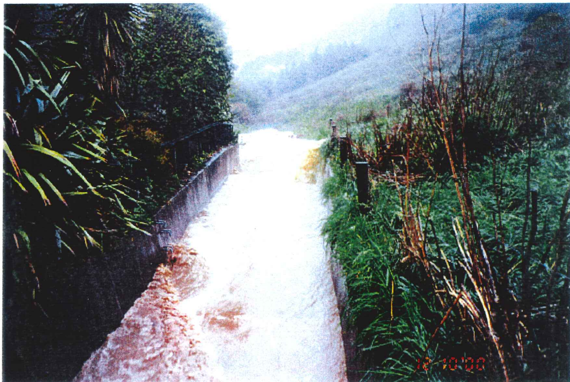
Sibleys Drain, Bowenvale Avenue below flume 12 October 2000
