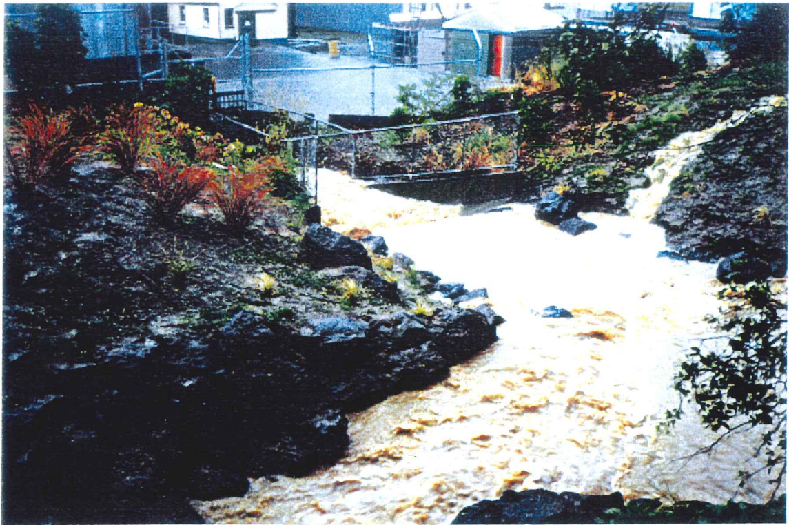
Typical hill waterway pipeline inlet conditions during the storm
