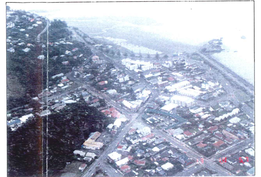
OVERVIEW OF FLOODED AREA
