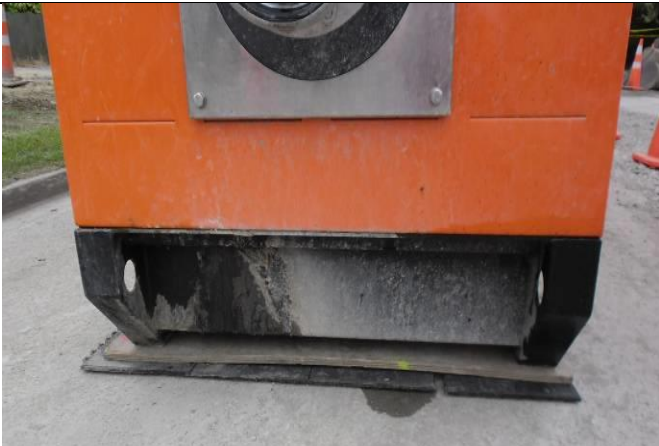
Figure 33: Noise Mitigation: Foam Mat and Plywood (to stop compression of foam)
