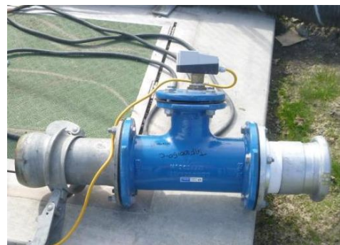
Figure 23: Flow Switch Unit for Discharge Pipe
