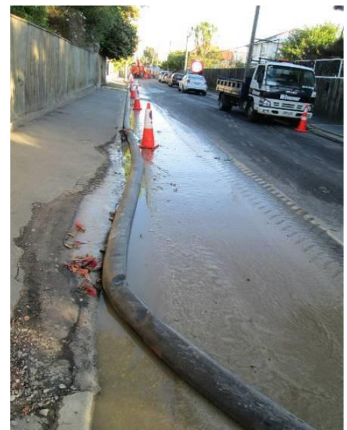
Picture 2: Wastewater sludge on a street following an overflow.
