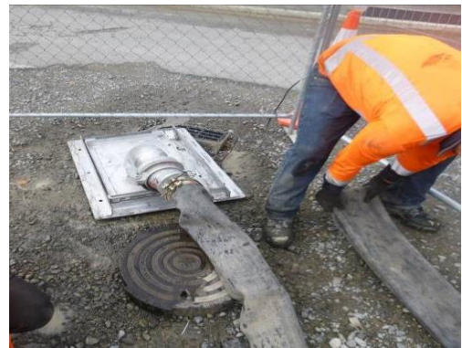
Figure 36: Manhole cover: Steel
