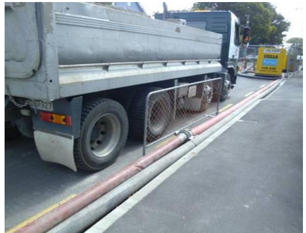
Figure 11: Traffic protection for pipes
