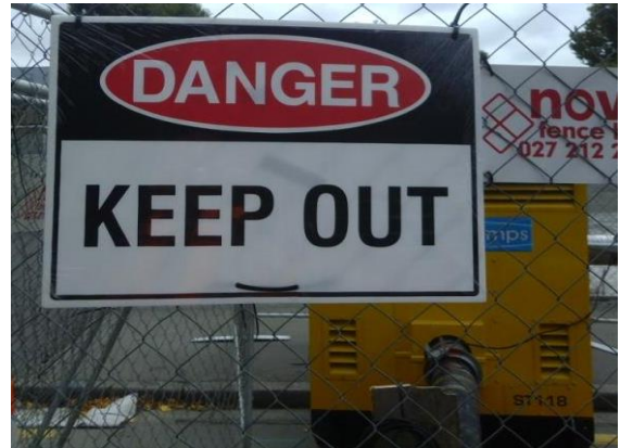
Figure 27: Danger Keep Out Signs
