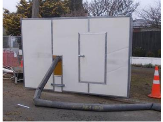
Figure 32: Noise Mitigation: Sound box
