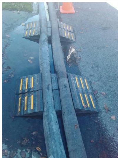
Figure 39: Pipe Protection: Ramps in front driveways
