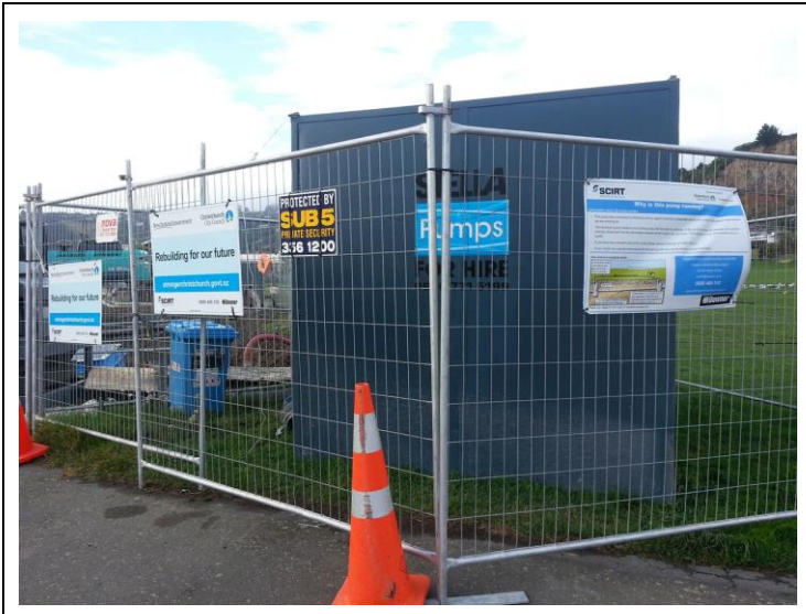
Figure 16: Locked site fencing around pump
