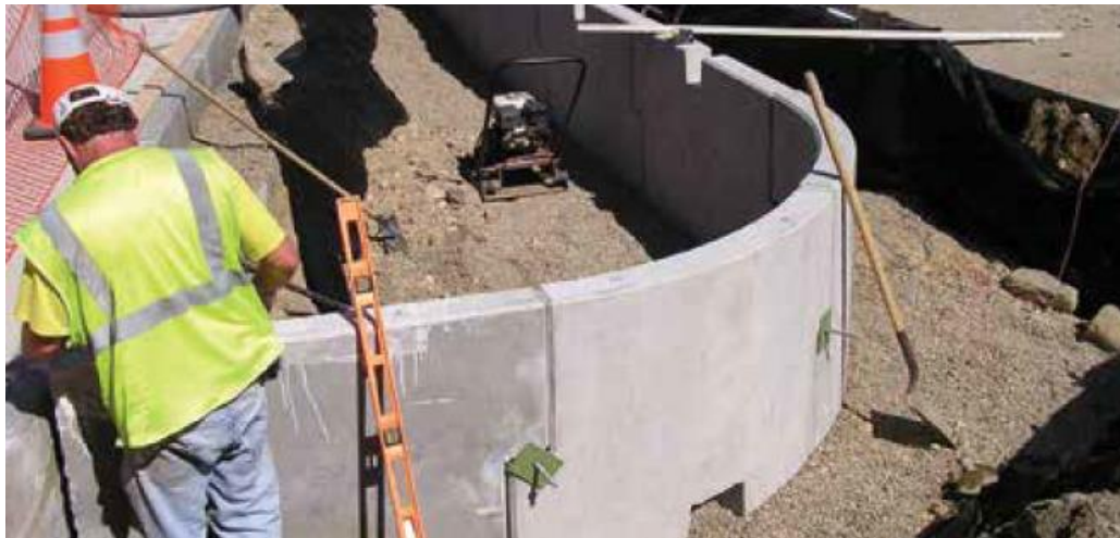
Figure 21 Precast concrete walls allow for fast installation
