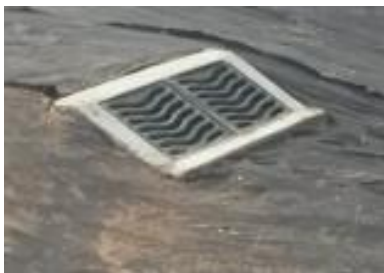
Figure 11 Double sump on batter slope overflow
