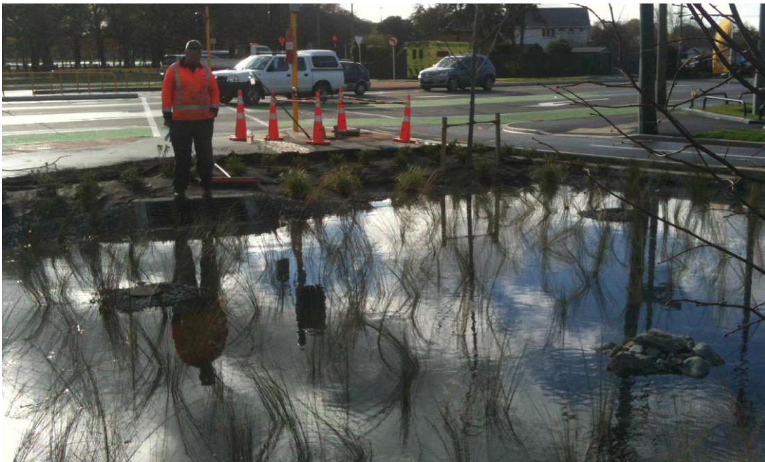
Figure 30 Grove Rd rain garden during infiltration testing
