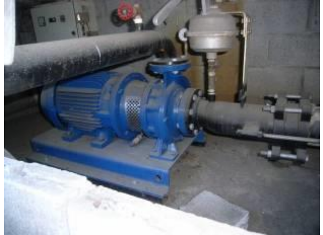
Pump and Motor on Irrigation System
