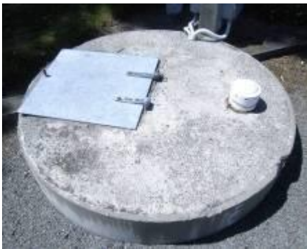
Wastewater Tank/Pump Chamber
