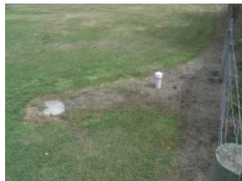
Buried Septic Tank. Vent and Access exposed.
